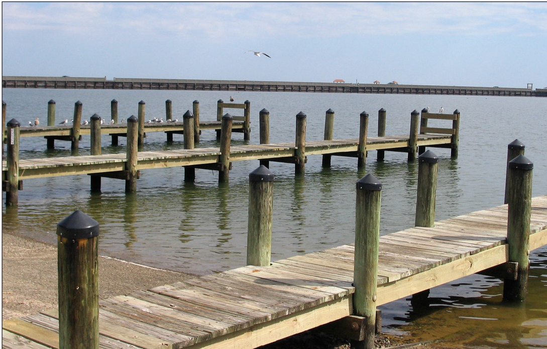
Figure 15. Wood immersed or partially immersed in seawater, such as these marine piles, is pressure-treated with increased retentions of chromated copper arsenate, ammoniacal copper zinc arsenate, or creosote to prevent attack by marine borers.
