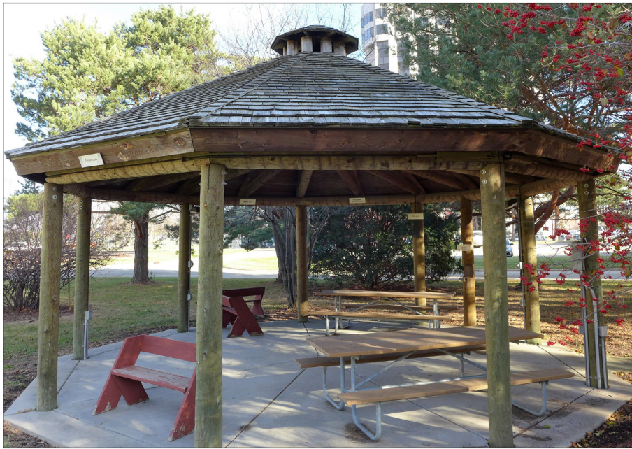
Figure 9. Round building poles and posts are structurally critical and pressure-treated to meet AWPA Use Category 4B.
