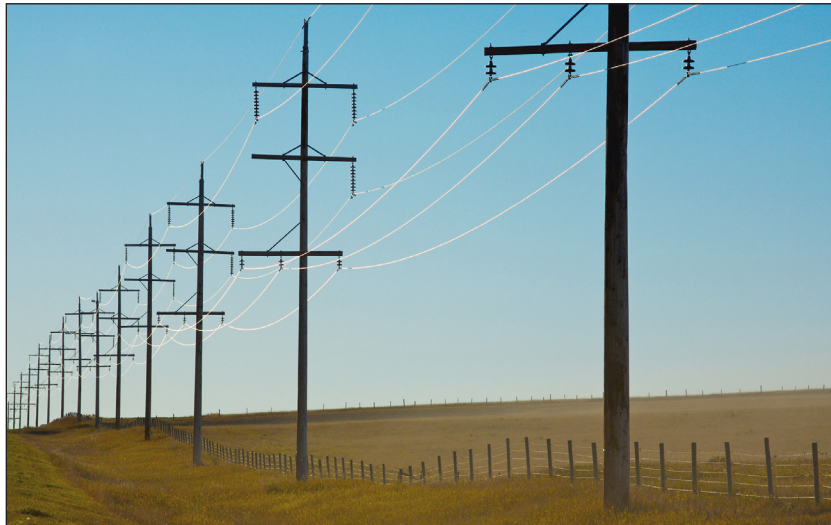
Figure 10. Pressure-treated poles are widely used to support transmission and distribution of electricity.
