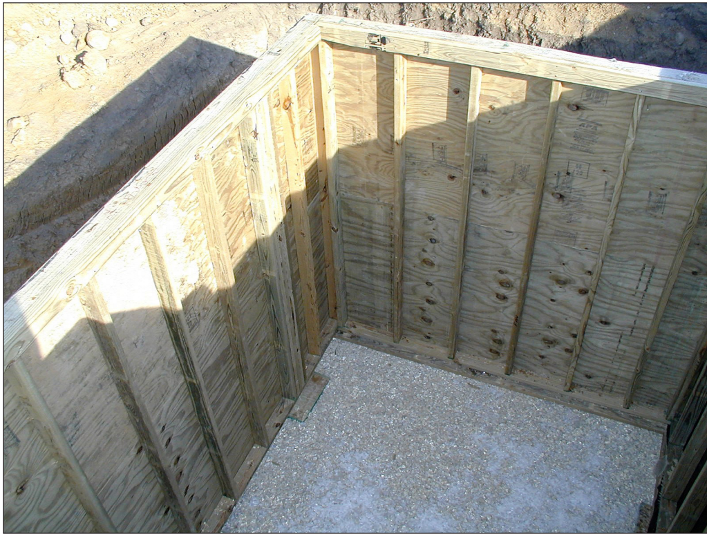
Figure 14. Lumber and plywood used for permanent wood foundations is structurally critical and is treated to meet AWPA Use Category 4B.
