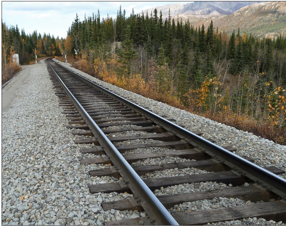
Figure 3. Creosote is often used for pressure treatment of railroad ties.
