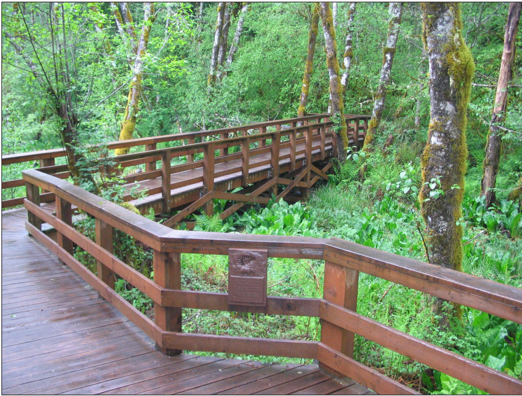
Figure 26. This wetland boardwalk in Oregon was part of a study to evaluate the leaching and aquatic impacts of treated wood used in sensitive environments.
