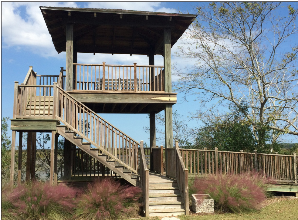
Figure 8. Pressure-treated lumber and sawn timbers are used in a wide range of structures.
