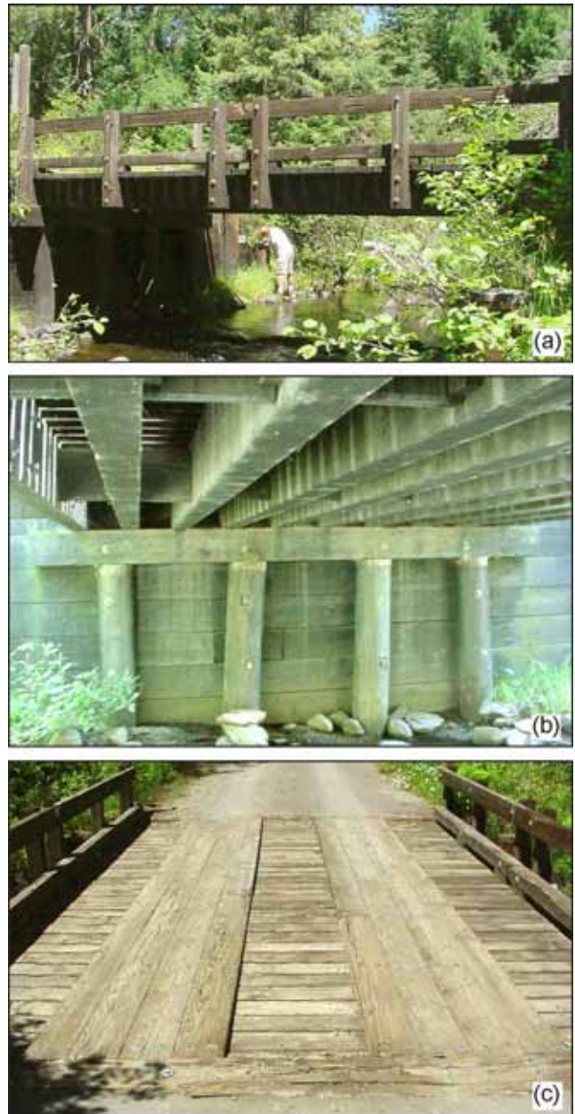
Figure 1—Typical single-span girder timber bridge: (a) side view, (b) structure, (c) deck.
