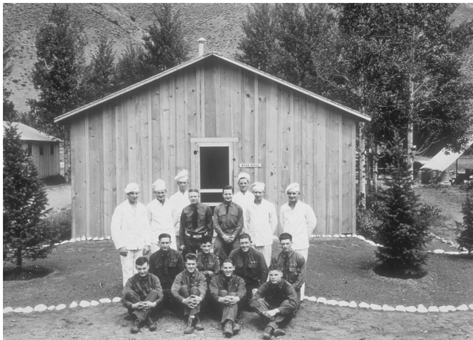
Front of Unknown CCC Camp Mess Hall
