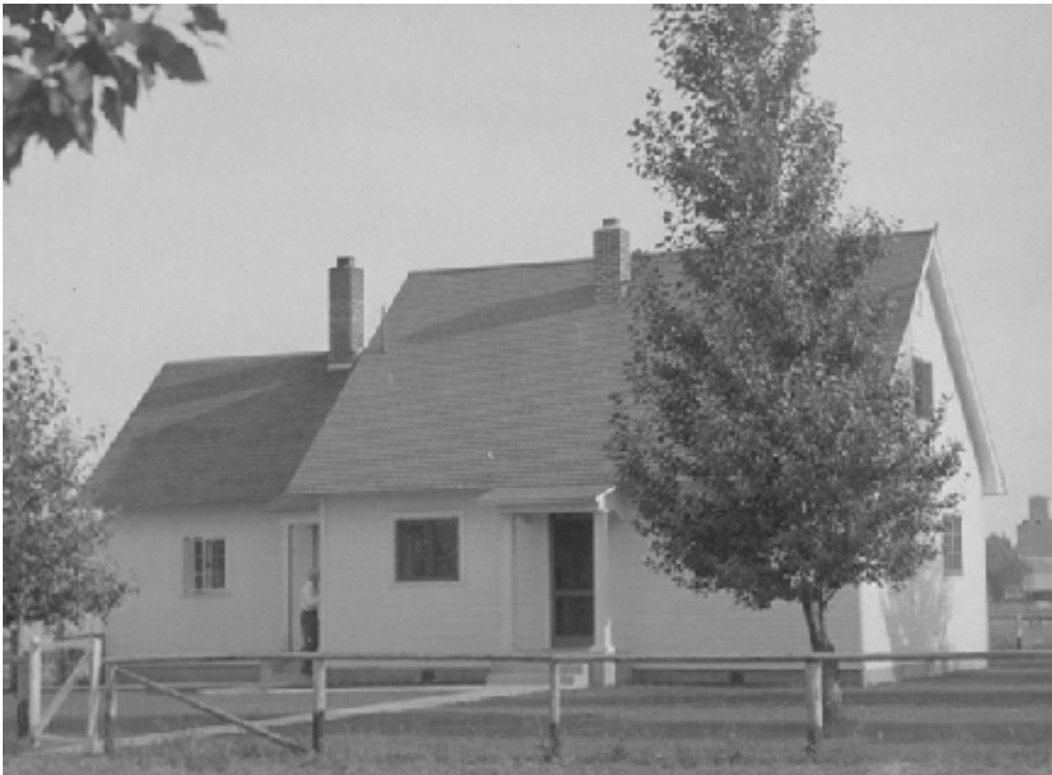
Fairfield Ranger Station, n.d.
