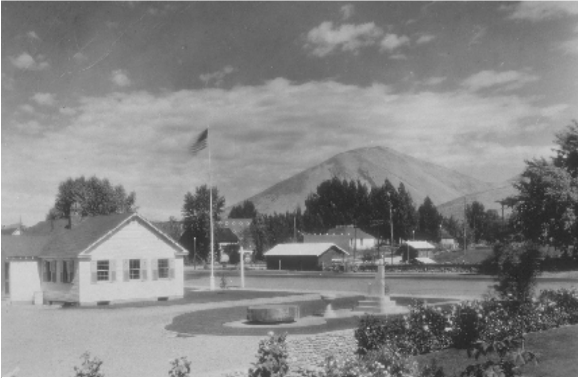
Supervisor's Office from Rear, Hailey, Idaho, n.d.
