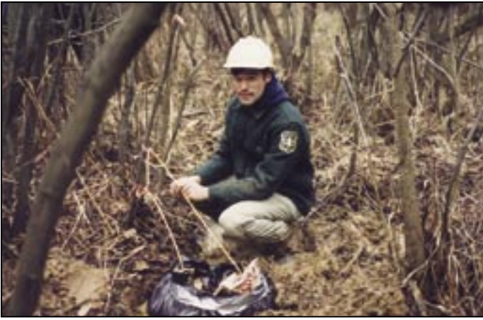
AN/FO is placed in a shallow hole.
