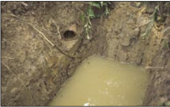
The core will crush buried drainage tiles.
