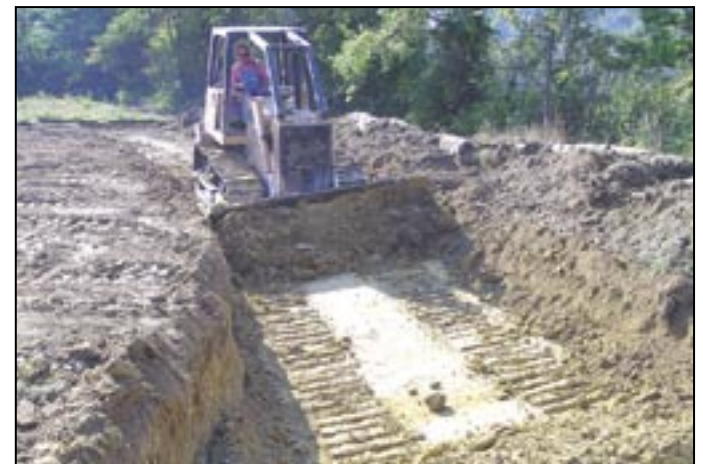
Core is located under the entire dam.
