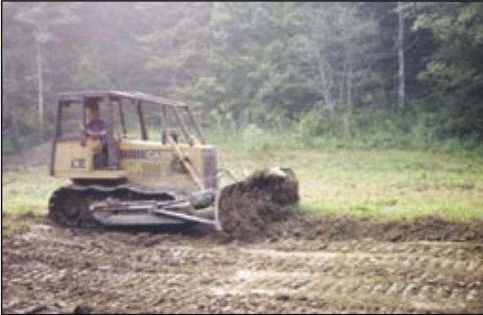
Remove and save topsoil.
