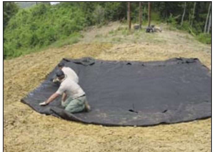
A liner is placed in the depression.
