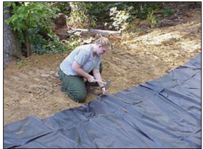
The liner is secured with stakes.
