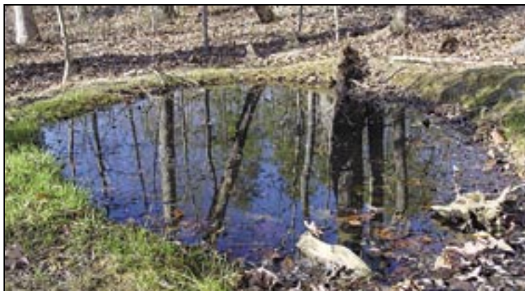
After placing the liner, they covered it with soil.
