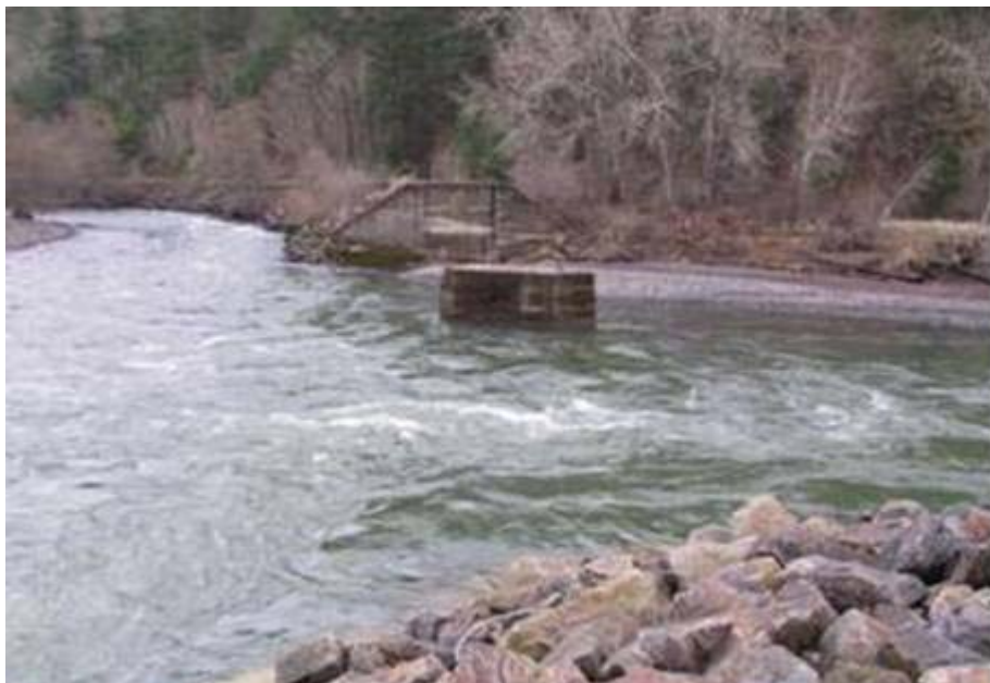
Figure 19: Remaining Structure from the Bridge over the Klickitat River at Suburbia.
