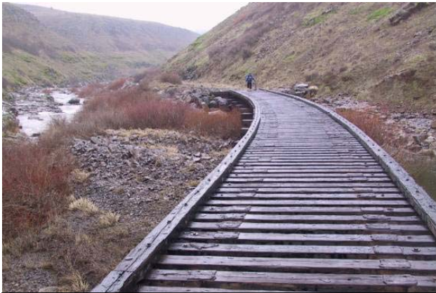
Figure 20: Typical Trestle in this Segment
