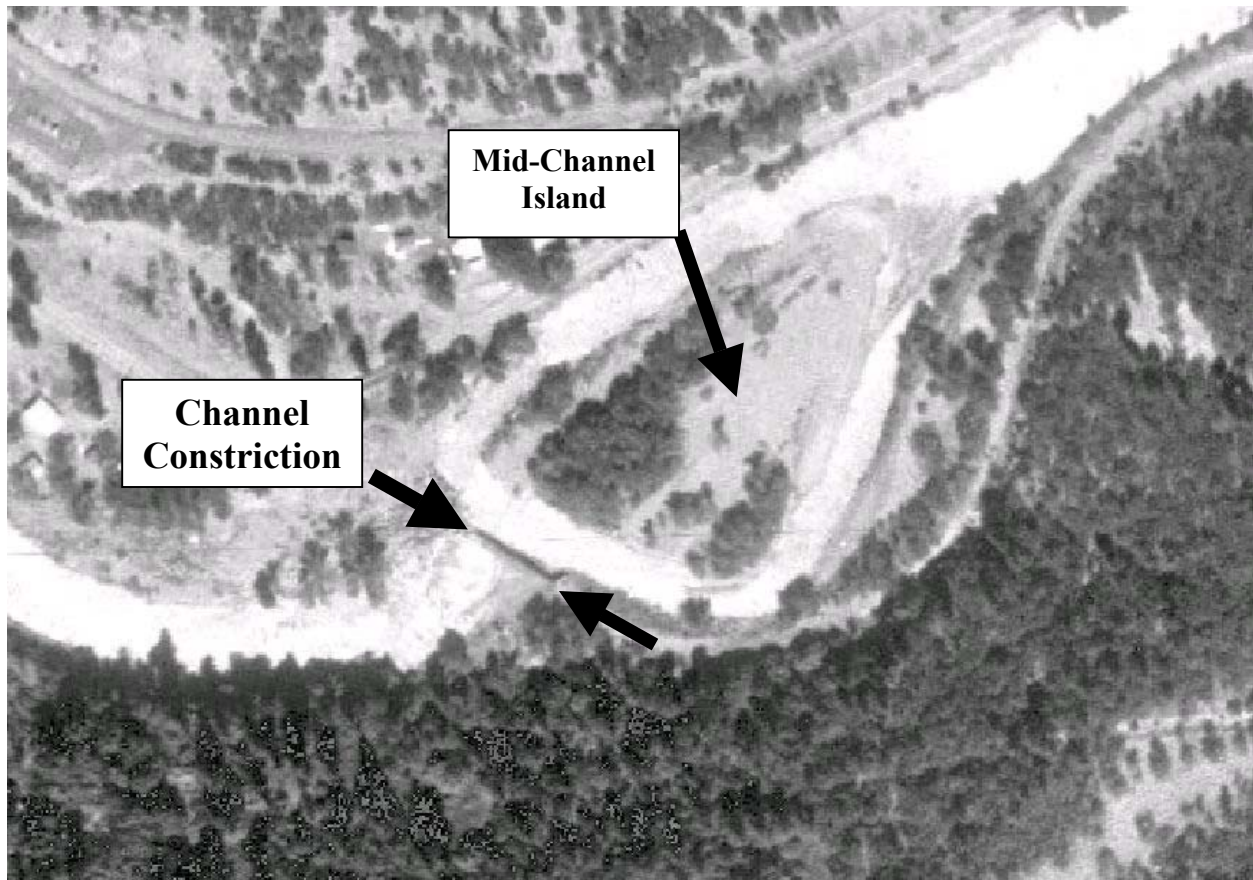
Figure 7: Air photograph showing constriction of the Klickitat River at Suburbia Bridge. This constriction has slowed water velocity and caused an island to form upstream of the bridge site.
