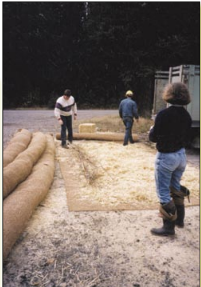
Figure 3–71—Erosion-control blanket logs are prepared by rolling out the erosion-control blanket, adding a layer of loose straw, and rolling a live fascine into the blanket.
