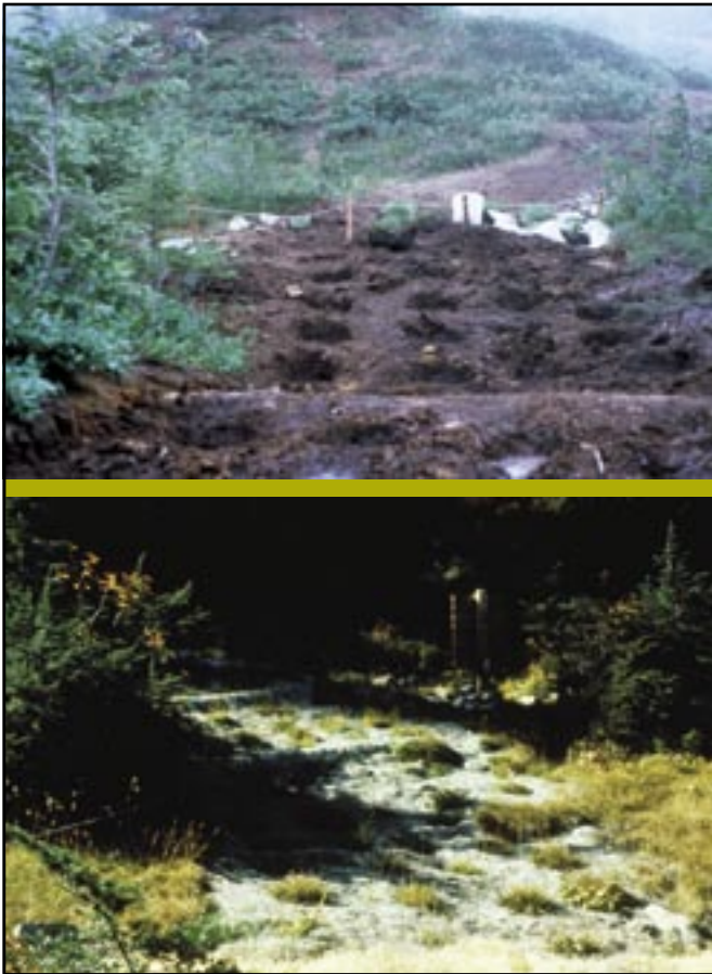
Figures 3–42a and 42b—This wide, severely eroded trail at Snow Lake in the Alpine Lakes Wilderness, WA (top), was brought back up to grade (bottom) by installing siltbars and adding many buckets of locally collected fill.
