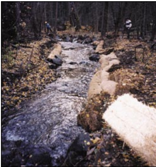
Figure 3–70—Live fascines rolled into erosion-control blankets can be used as “logs” to stabilize erosion along streambanks (Eubanks and Meadows 2002).
