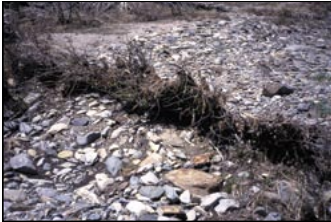
Figure 3–51—The live trench pack stabilizing this gully is one example of a living subsurface erosion control structure (Eubanks and Meadows 2002).
