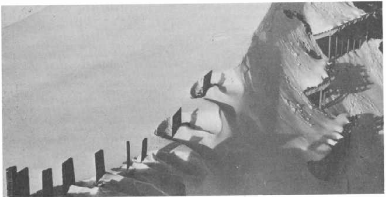
Figure 177.—Wooden eddy panels ( Kolktafeln ) on a slope (above) and a ridgecrest (below) above supporting structures. Note the disruption in the snow deposition caused by winds eddying around the baffles. (Photos by Frutiger)
