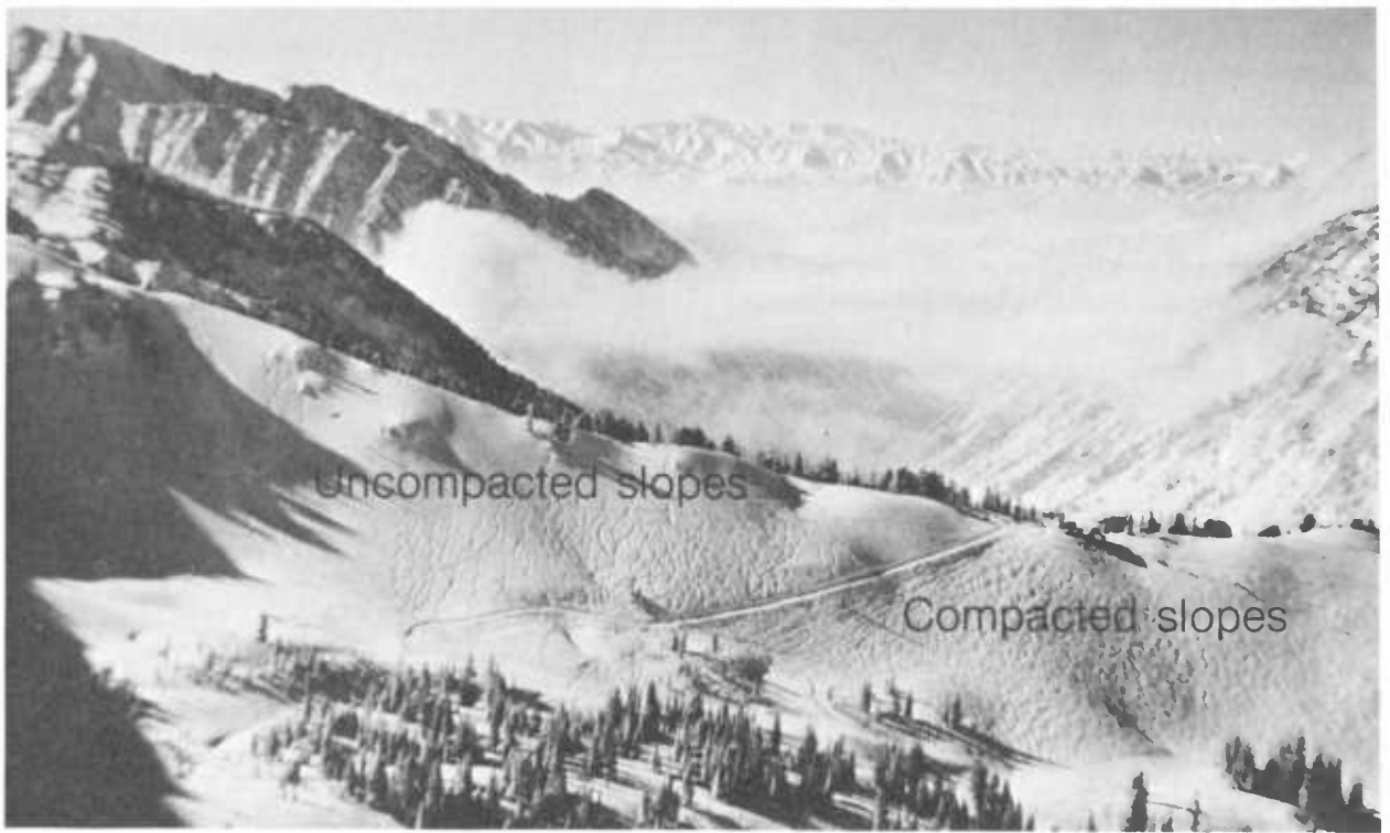
Figure 138.—Compacted and uncompacted slopes, side by side. Despite its steepness, the compacted slope (center and right) is a negligible avalanche problem. The uncompacted slopes (left) avalanche frequently.
