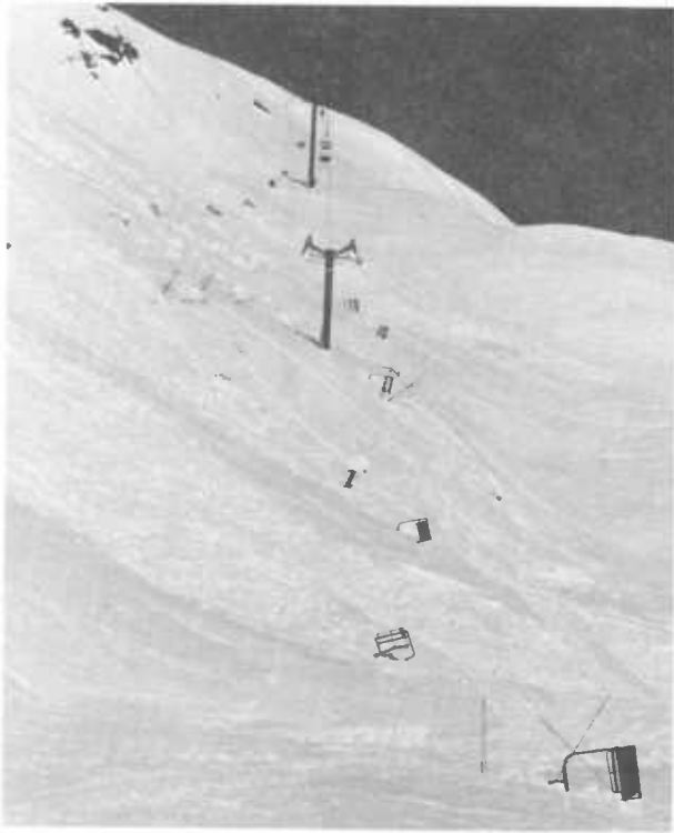
Figure 6.—Avalanche damage to a ski lift, Alyeska, Alaska, April 14, 1973. (Photo by O'Leary)
