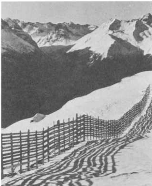
Figure 175.—Snowfences on a flat ridge to catch drifting snow before it goes over the steep rim where it might become an avalanche. Clüinas, Ftan, Switzerland. (Photo by Frutiger)
