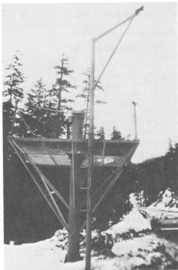
Figure 181.—75-mm recoilless rifle tower on Washington State highway. Winches are used to lift gun onto tower.
