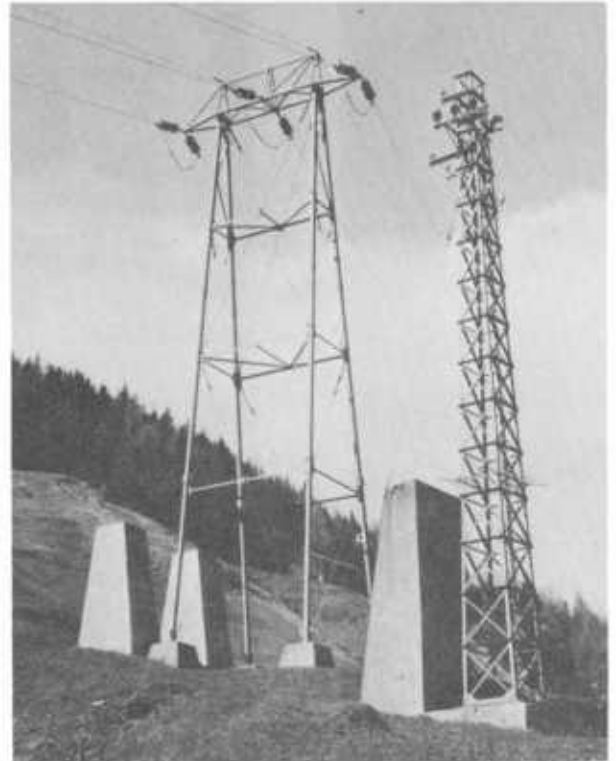
Figure 173.—Direct-protection structures: Left, a wedge-shaped concrete base for a high-voltage transmission tower located in an avalanche path (Beratungsstelle für Stahlverwendung 1962). Right, solid concrete blocks uphill from high-voltage towers. (Photo by Frutiger)
