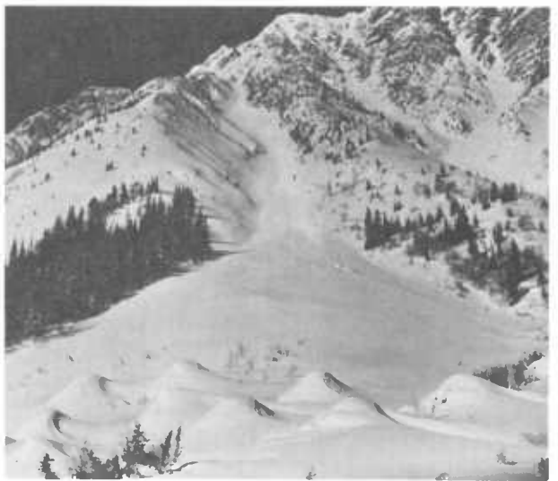
Figure 170.—Retarding structures used in avalanche paths: Left, mounds near Innsbruck, Austria. Right, mounds in the runout zone of Mt. Tupper Avalanche, Rogers Pass, B.C. (Photos by LaChapelle)
