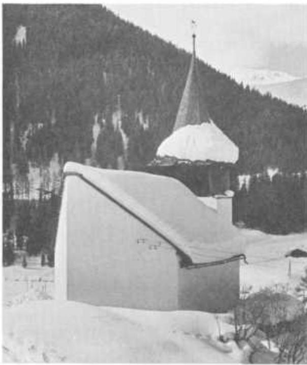
Figure 174.—Direct-protection structure: Special construction of the church at Davos-Frauenkirch, Switzerland, to withstand the impact of moving snow. (Photo by LaChapelle)
