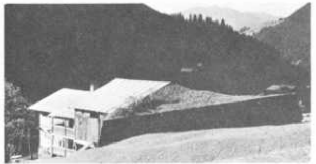
Figure 172.—Direct-protection structures: Top, earth ramps and wedges to protect buildings (Mellor 1968). Bottom, every house of the alpine settlement of St. Antönien has a mound of earth on the uphill side to protect it from avalanches. Gädmen-Matten-Meierhof, St. Antönien, Switzerland. (Photo by Frutiger)
