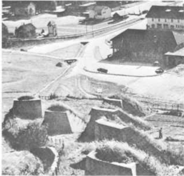
Figure 169.—Deflecting structures: Top, sketches of earth or masonry walls (Mellor 1968); bottom, concrete walls backfilled with earth to keep the avalanche that runs down the stream channel left of the fence from spreading to the right (Beratungsstelle für Stahlverwendung 1962).
