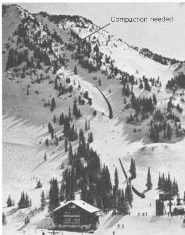
Figure 137.—An example of avalanche paths that should be thoroughly compacted beginning with the first snowstorm of the season. These paths threaten base facilities.
