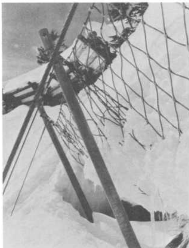
Figure 168.—Snow nets are flexible supporting structures. The triangular-shaped nets of wire rope are hung on tubular steel posts. Kneugrat, Braunwald, Switzerland (Frutiger and Martinelli 1966).
