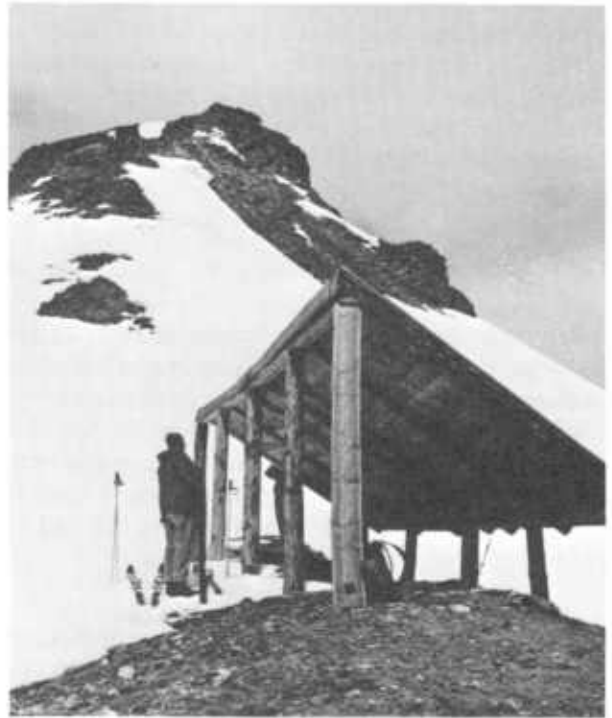
Figure 178.—Two types of sloping wind baffles used to prevent cornices: Left, pulpit used to carry wind and snow beyond the usual accumulation area. Right, jet roof that deflects wind down the lee slope so a cornice cannot form. (Photo by Frutiger)
