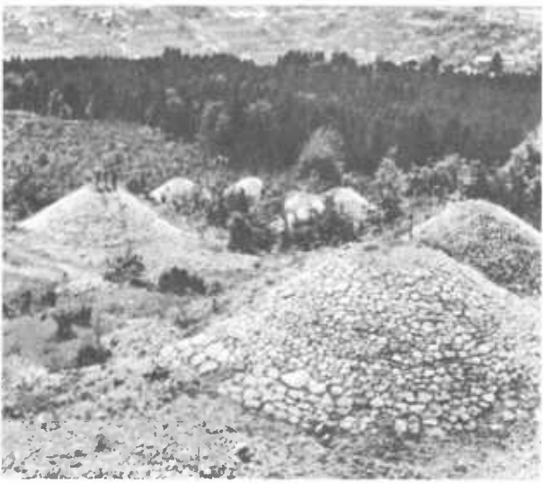
Figure 170.—Retarding structures used in avalanche paths: Left, mounds near Innsbruck, Austria. Right, mounds in the runout zone of Mt. Tupper Avalanche, Rogers Pass, B.C. (Photos by LaChapelle)
