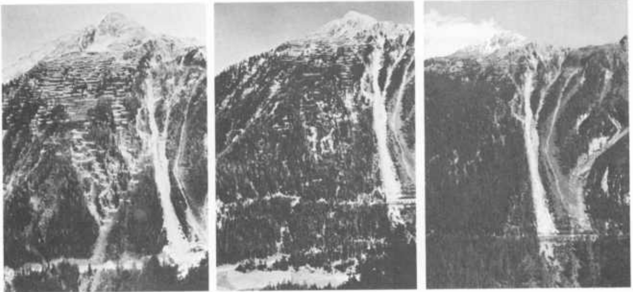
Figure 179.—The results of reforesting an avalanche path about 2.5 km south of Bergün on the Albula route of the Rhätische Bahn Grison, Switzerland. Left picture was taken in 1907; middle in 1938; right in 1957. A gallery 117 m long was built over the railroad at the foot of the right avalanche path. More than 10 km of retaining walls were built above timberline and over much of the rest of the mountain, then trees were planted. (Photos from Swiss Snow and Avalanche Research Institute with the permission of the Rhätische Bahn)
