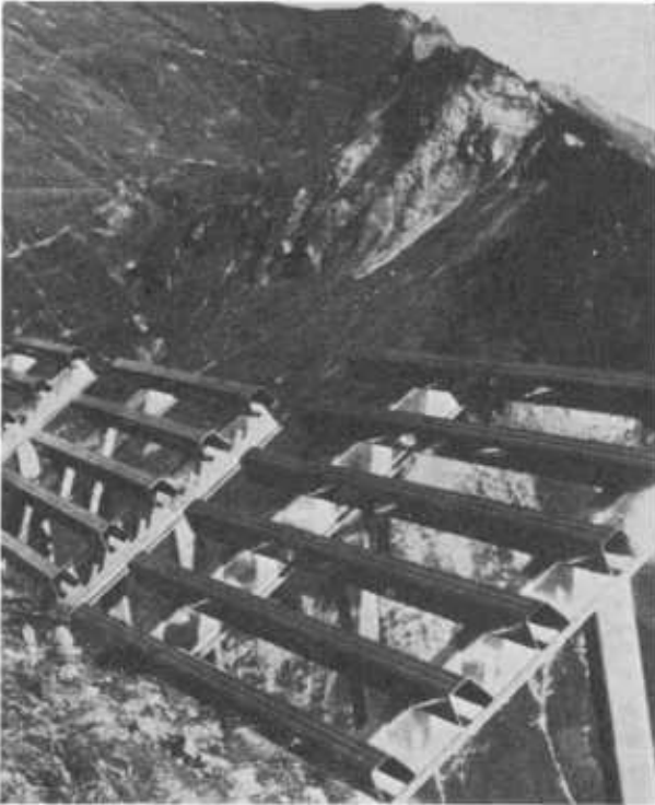
Figure 167.—Rigid supporting structures in the starting zone can be made from a variety of materials: Top left, aluminum frame and braces with wood crossbeams on the grate. Single snow bridges are no longer used; a continuous line of bridges is better. Mattstock Avalanche, near Amden, Switzerland (Wagner and Hopf 1959). Bottom left, aluminum snow bridges. Mattstock Avalanche, near Amden, Switzerland (Wagner and Hopf 1959). Top right, prestressed concrete snow bridge. Kühnihorn, near St. Antonien-Castels, Switzerland (Frutiger and Martinelli 1966).
