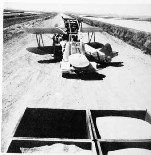
FIGURE 33.—Airplane being loaded with seed rice, with tanks used for soaking seed in the foreground, and ricefields ready to be seeded on each side of landing strip.
