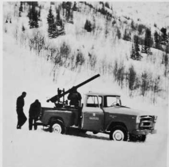
FIGURE 1.—105 mm. recoilless rifle mounted on a Forest Service truck. This is a highly mobile weapon for avalanche control.
