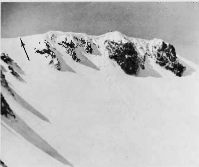
FIGURE 56.—Arrow points to cornice on Squaw Peak, controlled by drift fence. Compare absence of overhang with adjacent, uncontrolled cornices.
