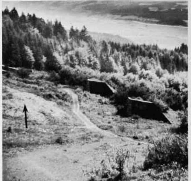
FIGURE 58.—Arzler Alm and the original system of avalanche breakers. Arrow indicated the mound of waste material which was the model for present-day design. Note natural reforestation behind the breakers.
