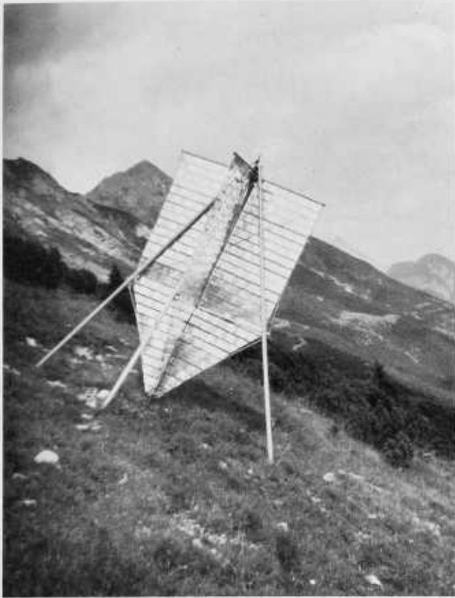
FIGURE 55.—Recently designed Austrian windbaffle, omnidirectional, tripod suspension, nose of baffle anchored to ground. The material is aluminum strips woven together with wire.
