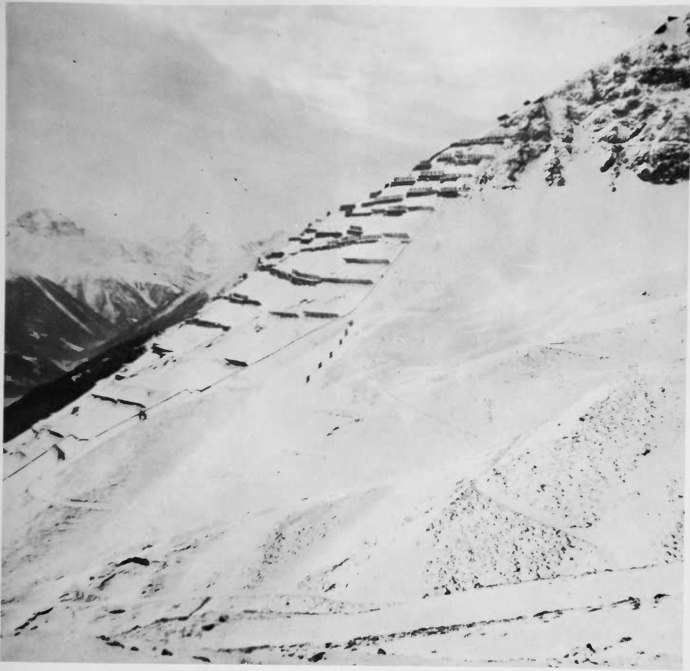
FIGURE 48.—A century of avalanche defense at Davos, Switzerland. Ancient masonry walls and terraces with Arlberg fences added later, and flanked by modern fences. The six dots near the center of the picture are wind baffles controlling an adjacent slide path.
