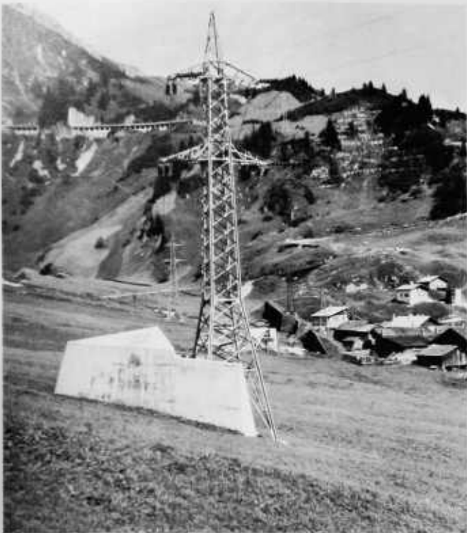
FIGURE 49.—Concrete bulkhead guarding an electric transmission pylon. Note diversion wall protecting houses to right, Arlberg fences above, and snowshed at upper left. Stuben, Austria.
