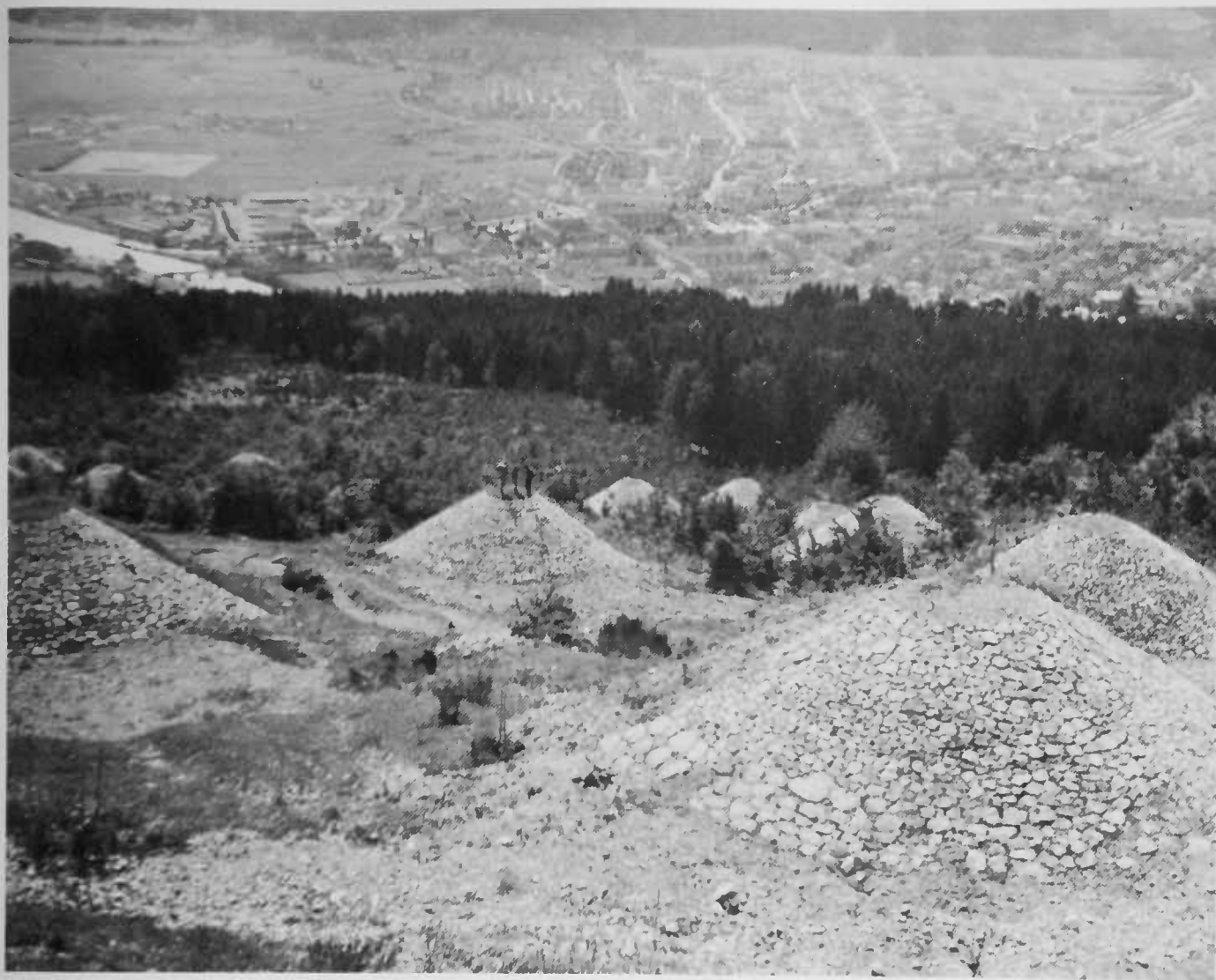
FIGURE 59.—Modern avalanche mound system, near Innsbruck, Austria.
