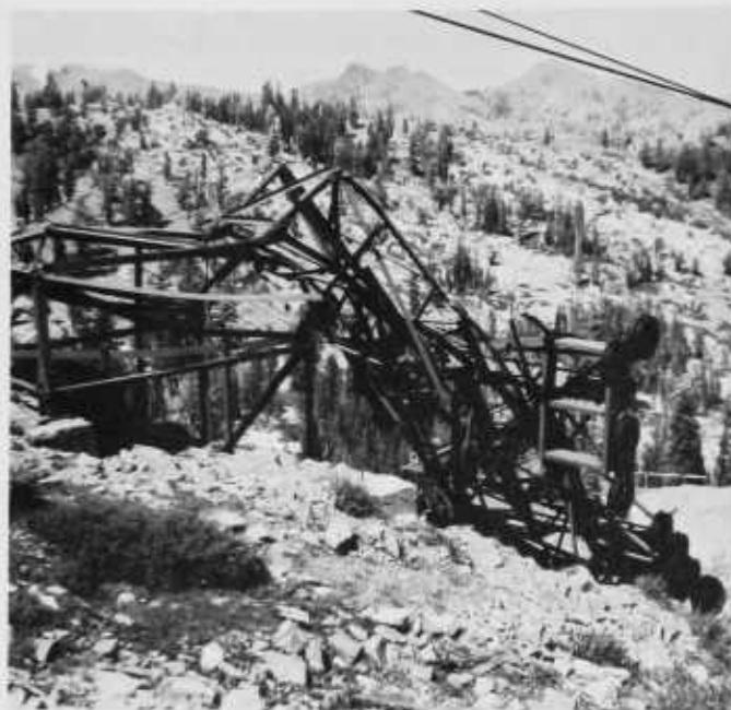
FIGURE 74.—Avalanche destruction of a lift tower.
