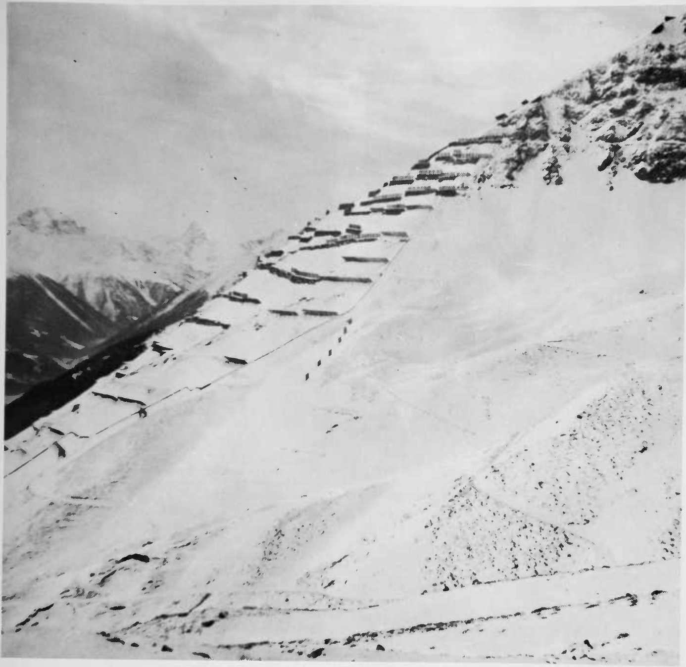
FIGURE 48.—A century of avalanche defense at Davos, Switzerland. Ancient masonry walls and terraces with Arlberg fences added later, and flanked by modern fences. The six dots near the center of the picture are wind baffles controlling an adjacent slide path. F-495212
