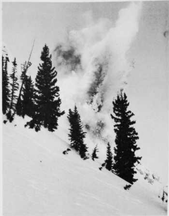
FIGURE 43.—Removal of cornice by a heavy charge of tetrytol.
