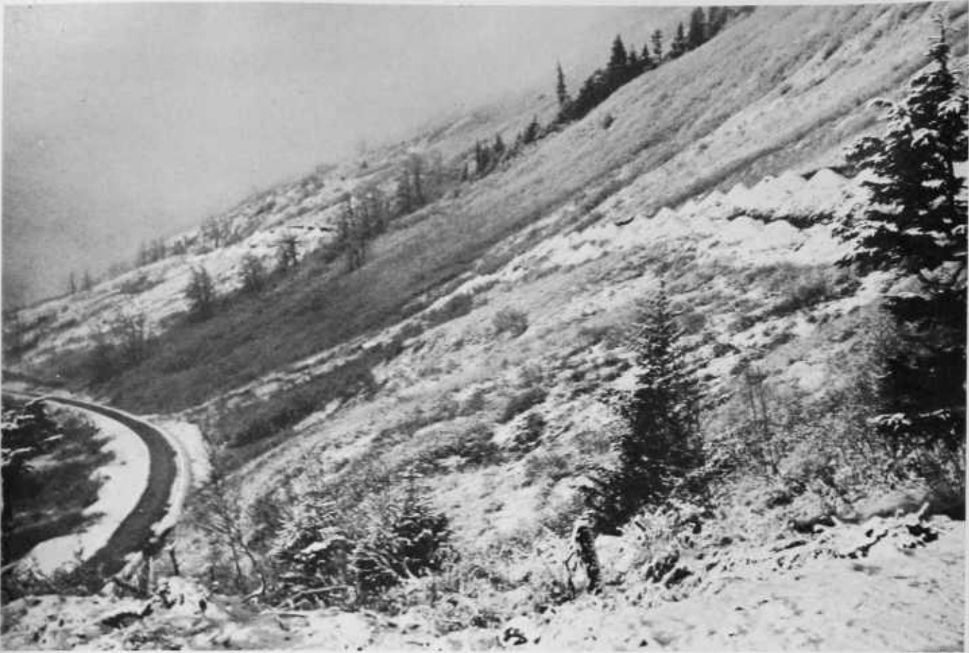
FIGURE 60.—Earth mounds used as avalanche breakers near Girdwood, Alaska. Though a transition zone is absent on this slope, these mounds have proved an effective defense against wet slides.
