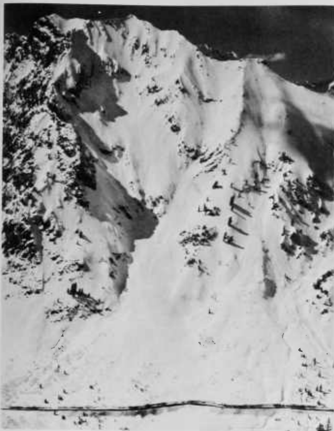
FIGURE 71.—An example of avalanche hazard. A major avalanche path, with vertical relief of nearly 4,000 feet, overhangs the access highway leading to a major ski resort. Protective measures used are road closures during high hazard, and artificial release of avalanches by artillery fire.
