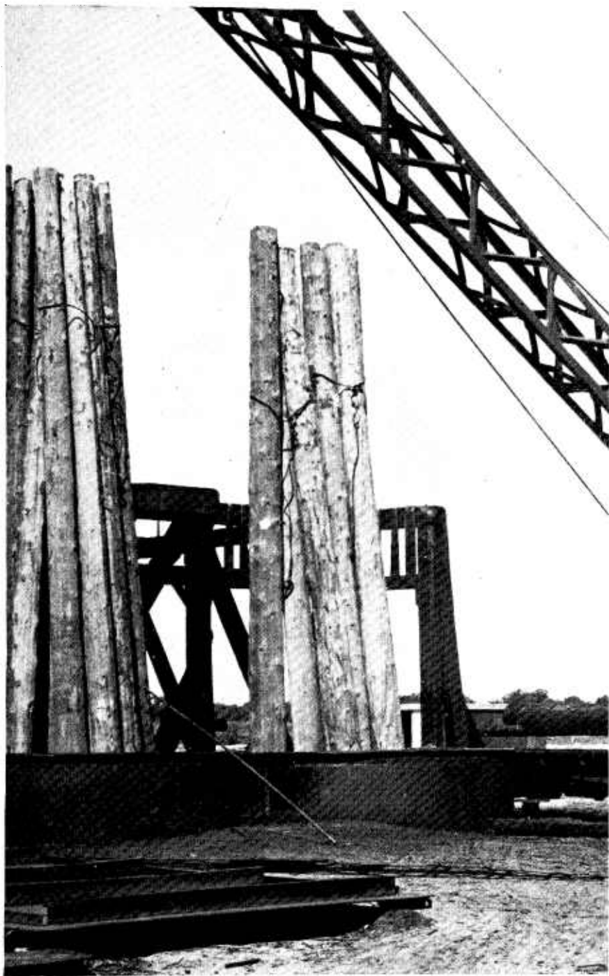
FIGURE 89.—Tanks for butt treatment of poles by hot-and-cold-bath process.
