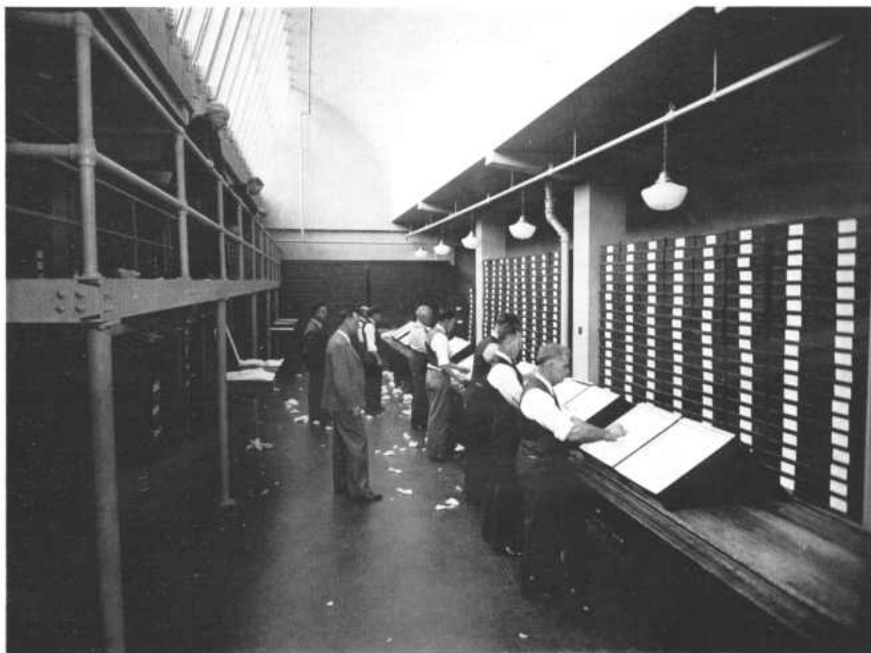
FIGURE 43.—One of the latest type of skylights developed for cotton classing rooms of the United States Department of Agriculture. The skylight in this room is 80 feet long, set facing north, with glass set at an angle of 72° from the horizontal (related to the latitude in which it is built), a concave reflecting surface opposite the skylight windows to diffuse the light, and no cross beams in the construction to throw shadows.
