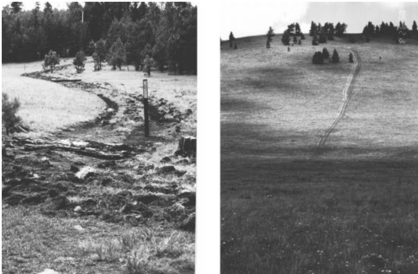
Figure 4.5: Unauthorized Roads on Forest Service Land
