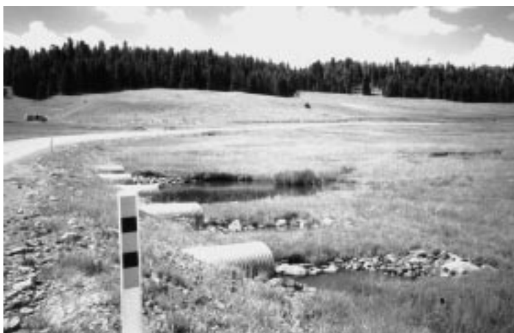
Road improvement to reduce streambank erosion. Multiple culverts employed to divert and slow flow.
