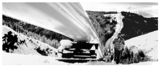
(3) An interstate system of piplines transports natural gas to local markets in the United States. This system is composed of over 300,000 miles of piping, not including local distribution lines. Many pipelines intersect at market centers that provide numerous routes to move gas to local markets, in addition to providing related services such as short-term gas storage and gas loaning.
