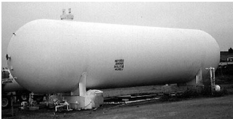
At the dealerships, the anhydrous ammonia is stored in pressurized "bullet" tanks. This bullet tank holds 30,000 gallons (about 77 tons).
