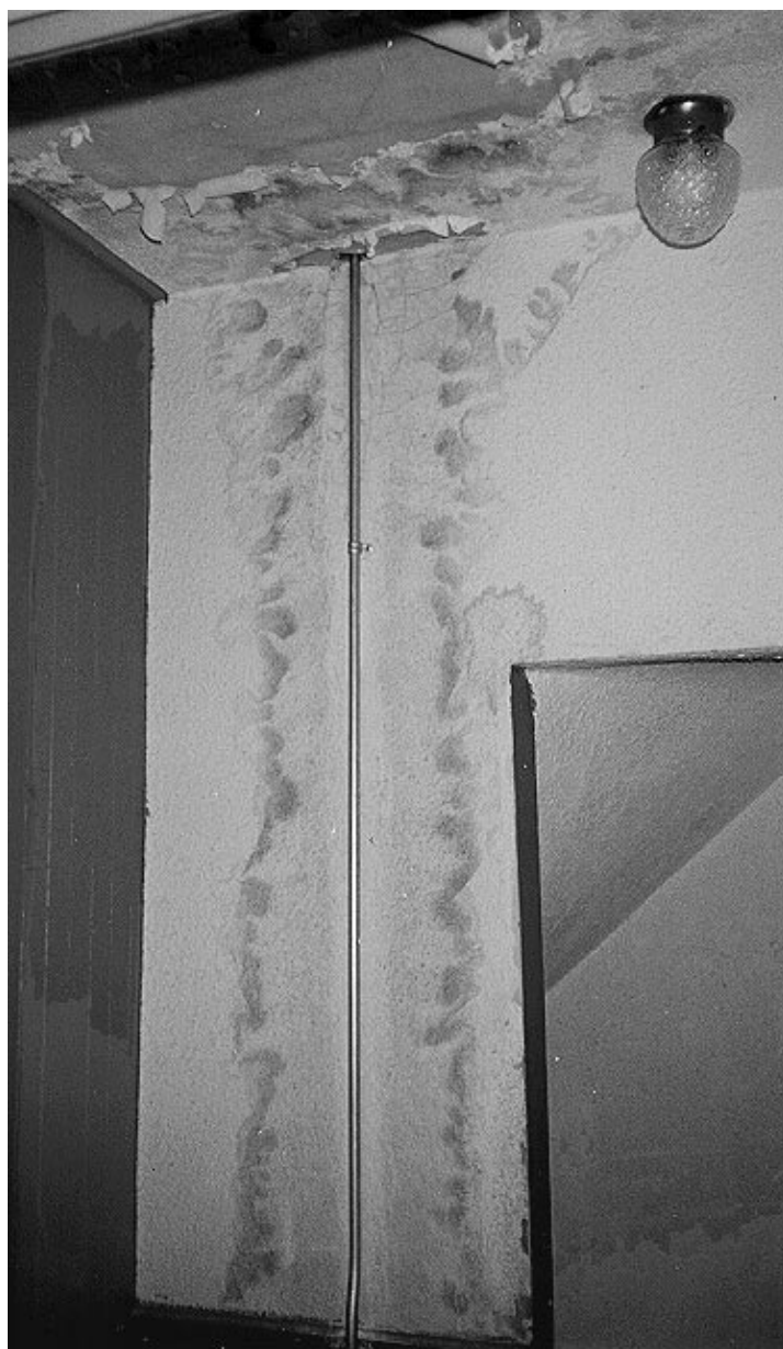
Extensive water damage resulting from a broken skylight
