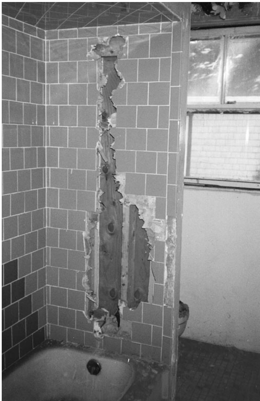
Figure 2: Copper Piping Ripped Out of Wall at an Improperly Secured Property
