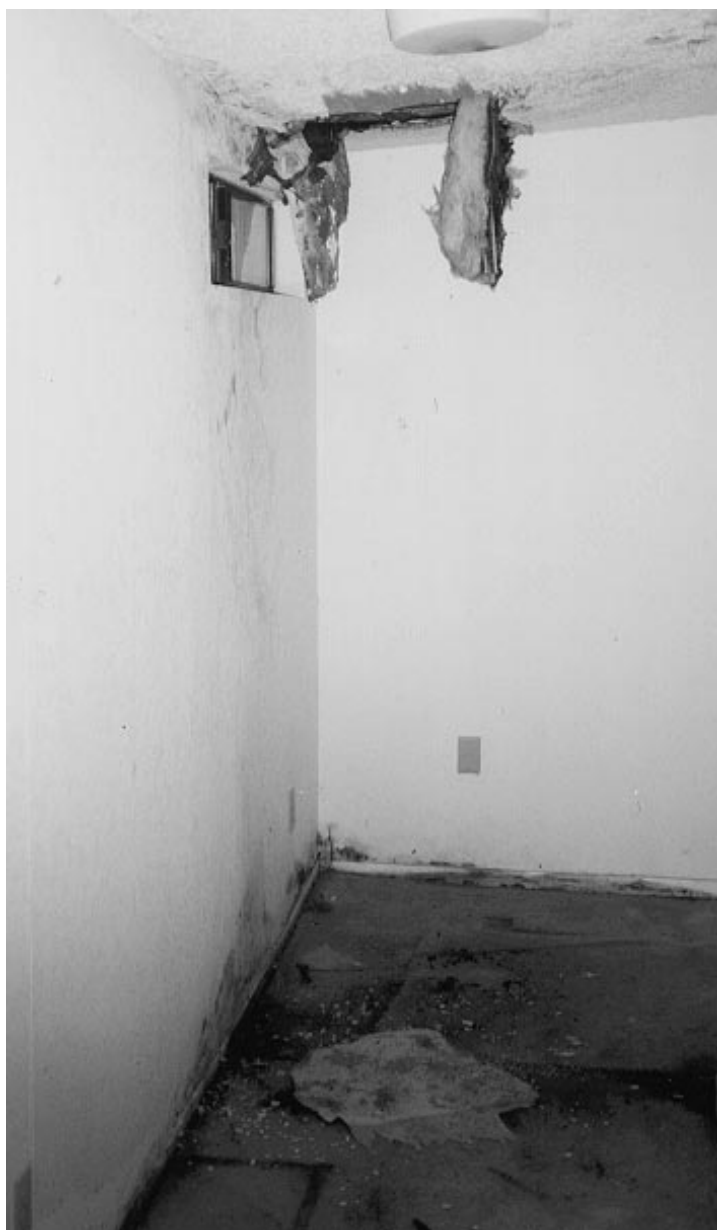
Water damage resulting from active roof leaks
