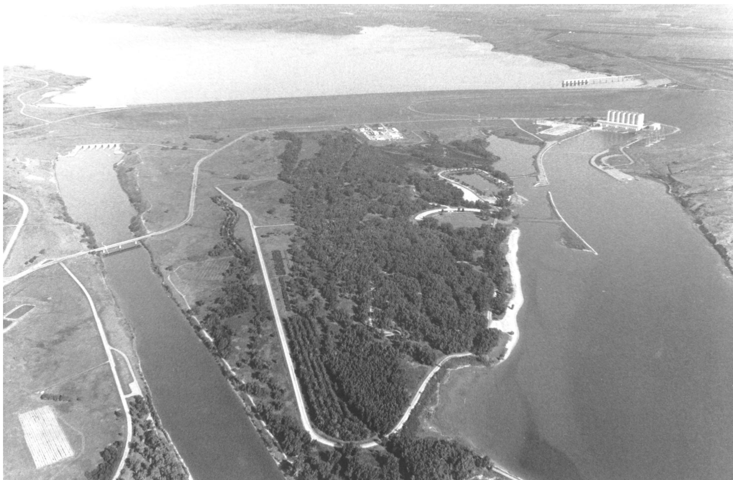
Figure 1: The Oahe Dam
