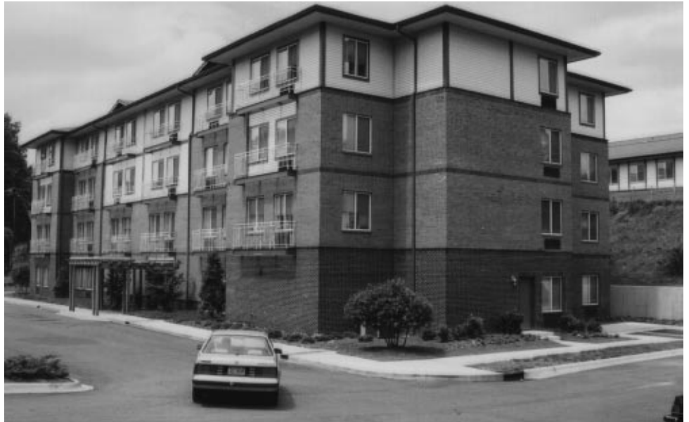
Figure I.5: Granville Plaza Section 202 Project, Winston-Salem, North Carolina
