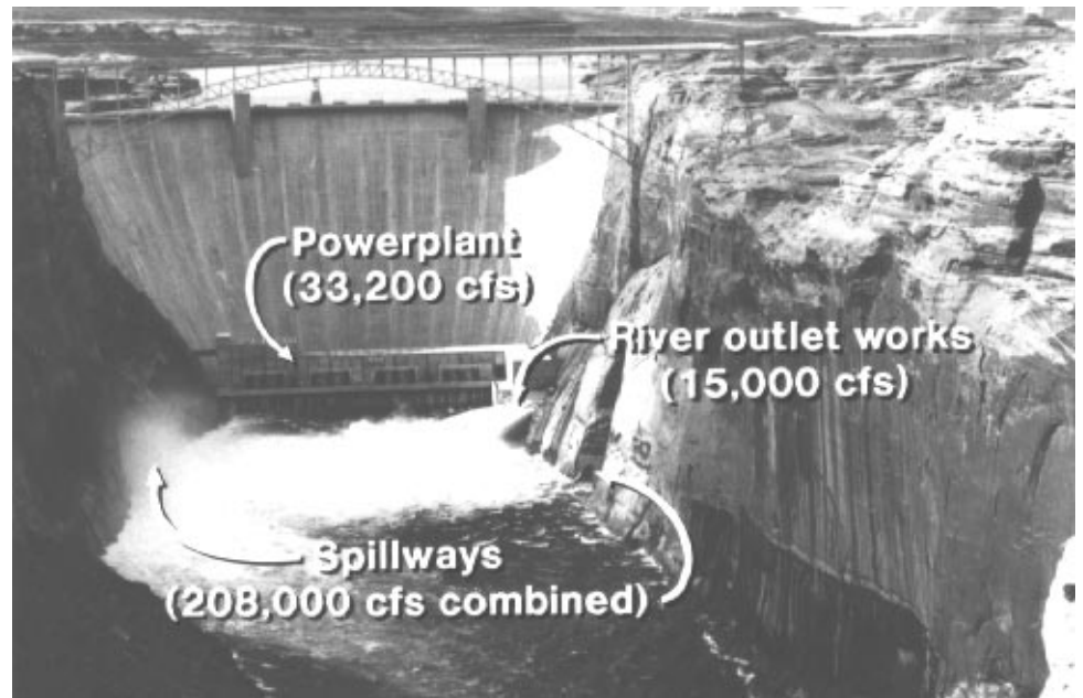
Figure 1.1: Water Release Capacities of the Glen Canyon Dam's Powerplant, Outlet Works, and Spillways
