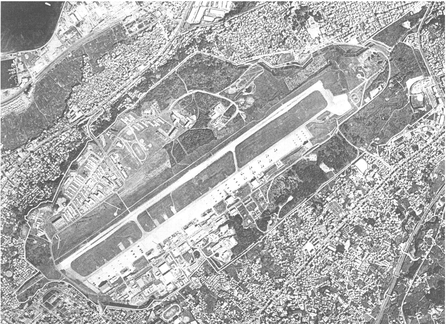
Figure 3.1: Aerial View of MCAS Futenma
