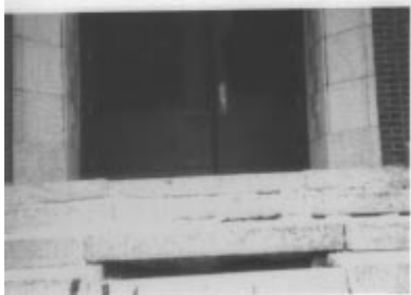
...Holes in Crumbling Front Steps Chicago High School
