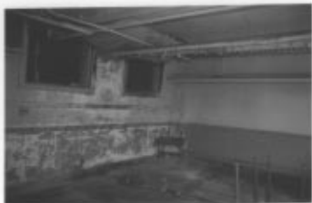
Basement Chicago Elementary School
