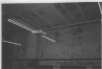
Peeling Lead-Based Paint, Burned Out Lights (Not Replaceable) Chicago Elementary School
