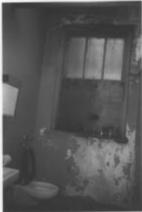
Student Bathroom Chicago Elementary School
