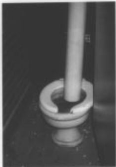
Toilet Used to Redirect Sewage From Broken Pipe in Wall District of Columbia High School
