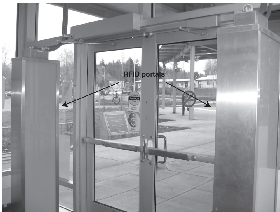
Figure 7b: RFID Portals Positioned Next to Exit Doors at the Blaine-Peace Arch POE in Washington State
