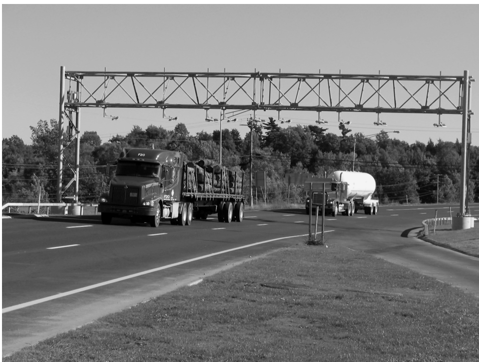
Figure 7a: Metal Gantry with RFID Readers and Antennas at the Thousand Islands Bridge POE, Alexandria Bay, New York
