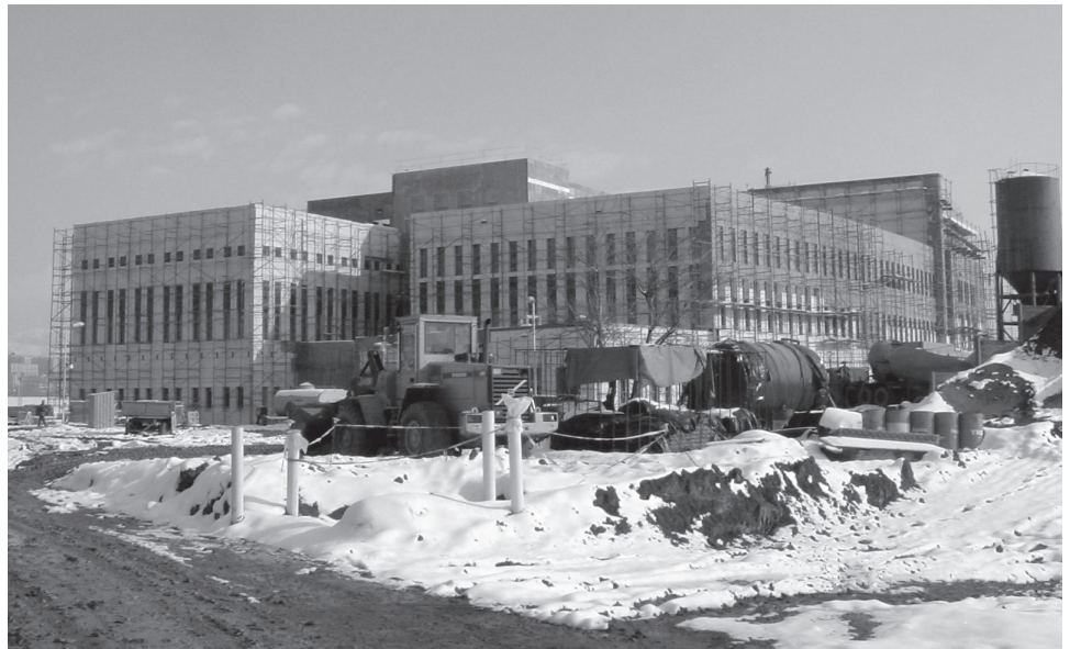
Figure 2: Construction of the Standard-design New Embassy Compound in Tbilisi, Georgia
