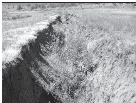
Irrigation Ditch in Need of Reshaping
