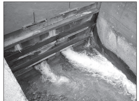
Leaking Check Gate
