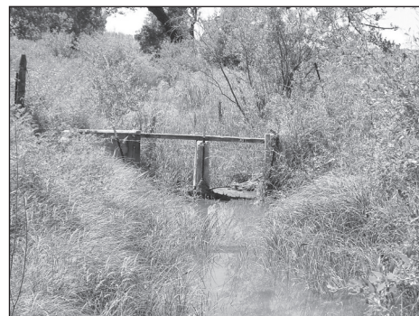
Overgrown Vegetation Around Dilapidated Irrigation Check Structure
