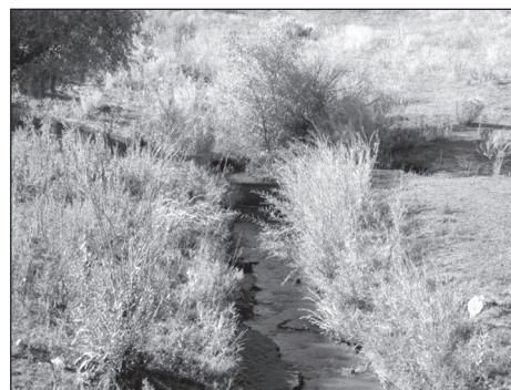
Overgrown Vegetation in Irrigation Ditch
