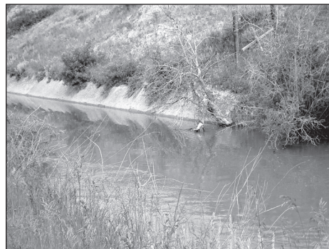
Source: GAO. Deteriorating Canal Lining
