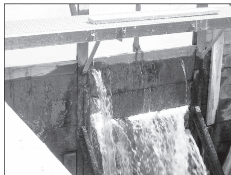
Leaking Check Gate
