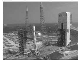
Delta IV East Coast Launch Site, Space Launch Complex 37, Cape Canaveral Air Force Station, Florida
