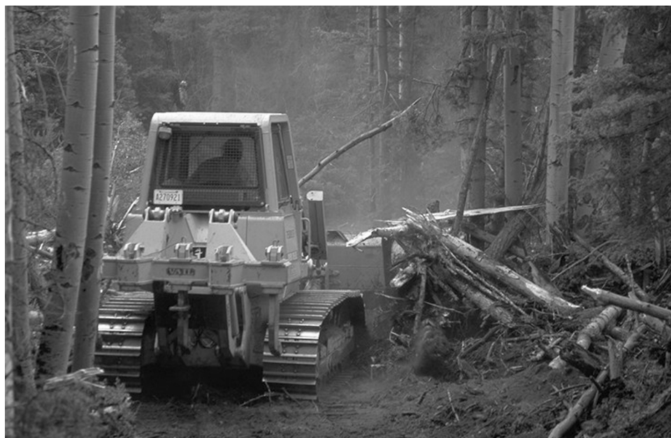
Figure 7: Bulldozer Piling Thinned Trees (Machine Piling)
