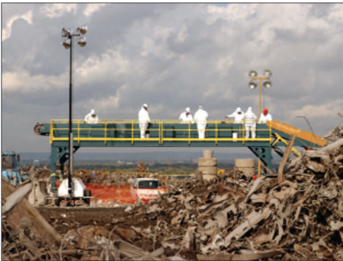
Figure 4: Debris Screening and Inspection Operations
