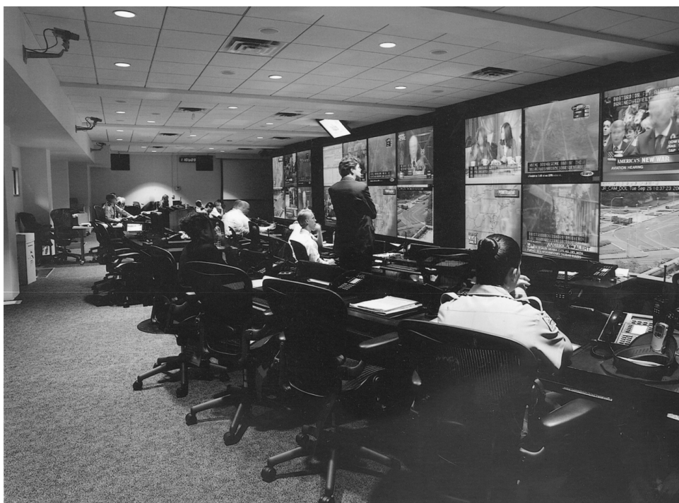
Figure 3: A CCTV Control Room
