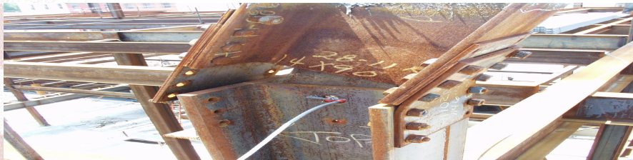
A close-up of one of the steel trusses involved in the collapse.
