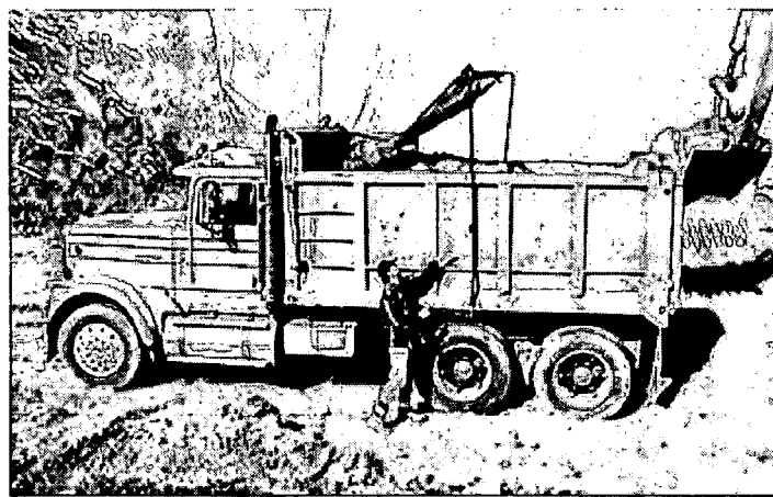
Excavation equipment working on the construction site.
