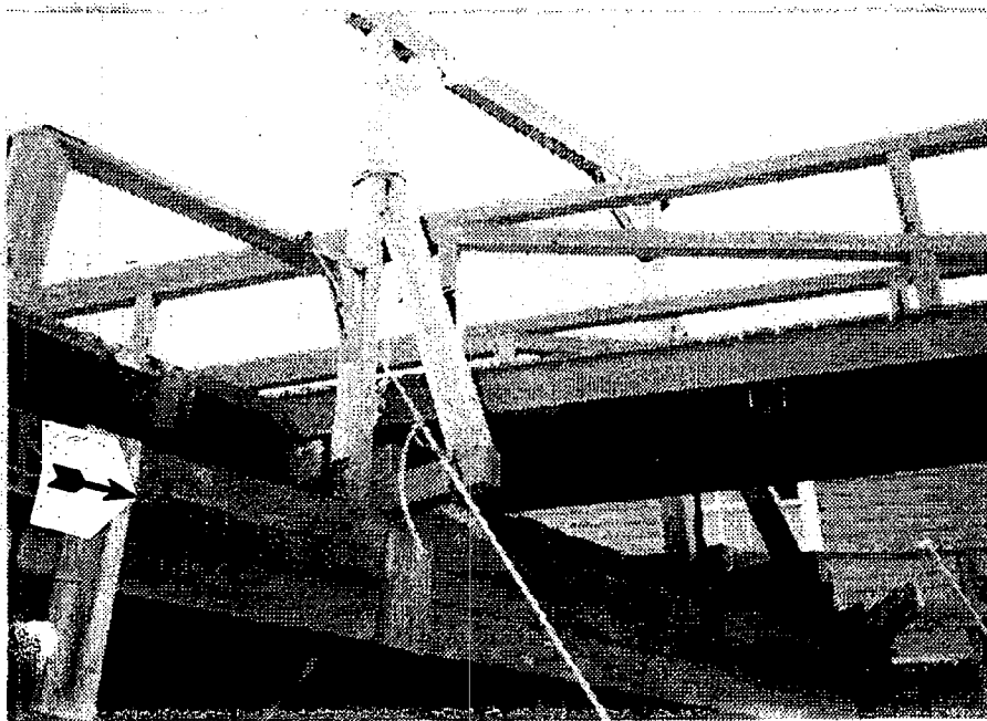
Town float, some beams showing signs of decay.
