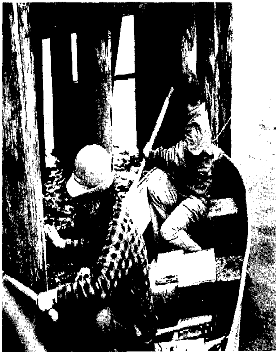
Figure 13 Consultants taking wood borings of the piles to determine the structural condition of the North Pier
