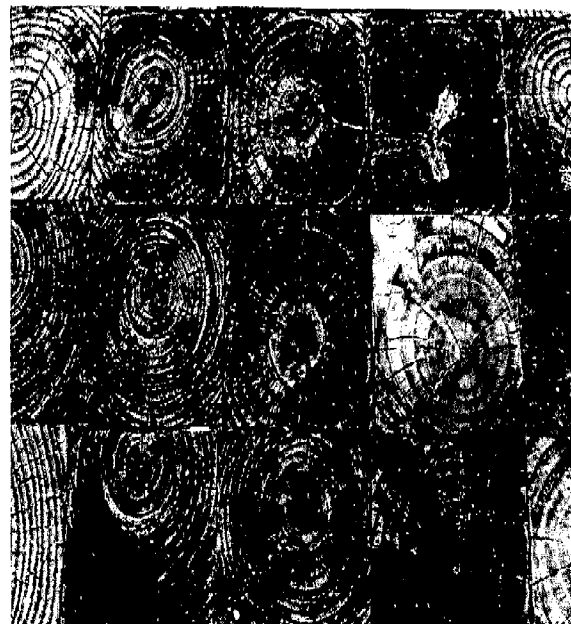
Figure 25 Nautical wood block paving pattern at Annapolis City Pier.
