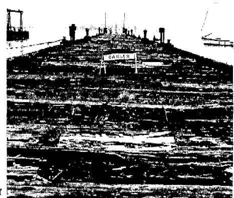
Figure 15 Deteriorated timber deck on South Pier
