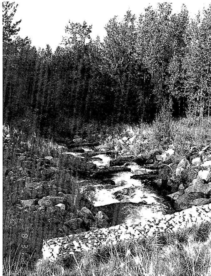
Plate 34. Rabbit Creek fish pass in 1993. The structure continues to function as intended, although no fish were observed there. Other obstacles downstream may be interfering with fish migration through this project area.
