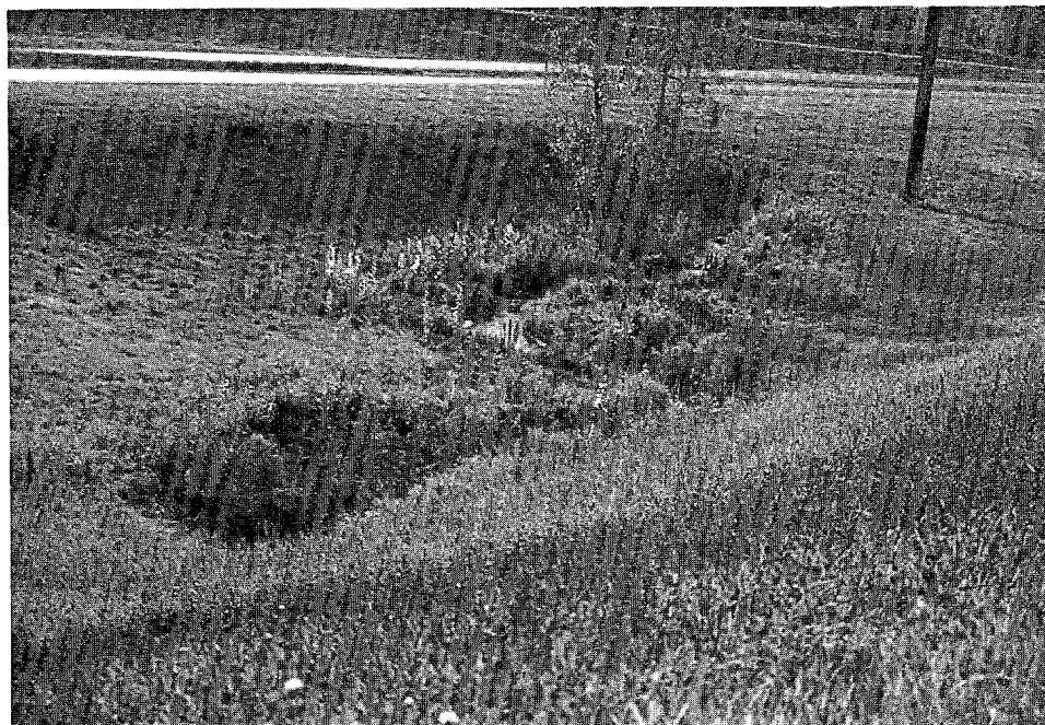
Plate 10. Realigned section of Carrol Creek at the North Eagle River highway interchange (between the "A2" ramp and the highway, see Figure 5). Willow cuttings are persisting in this area more than in the other sections of the project.
