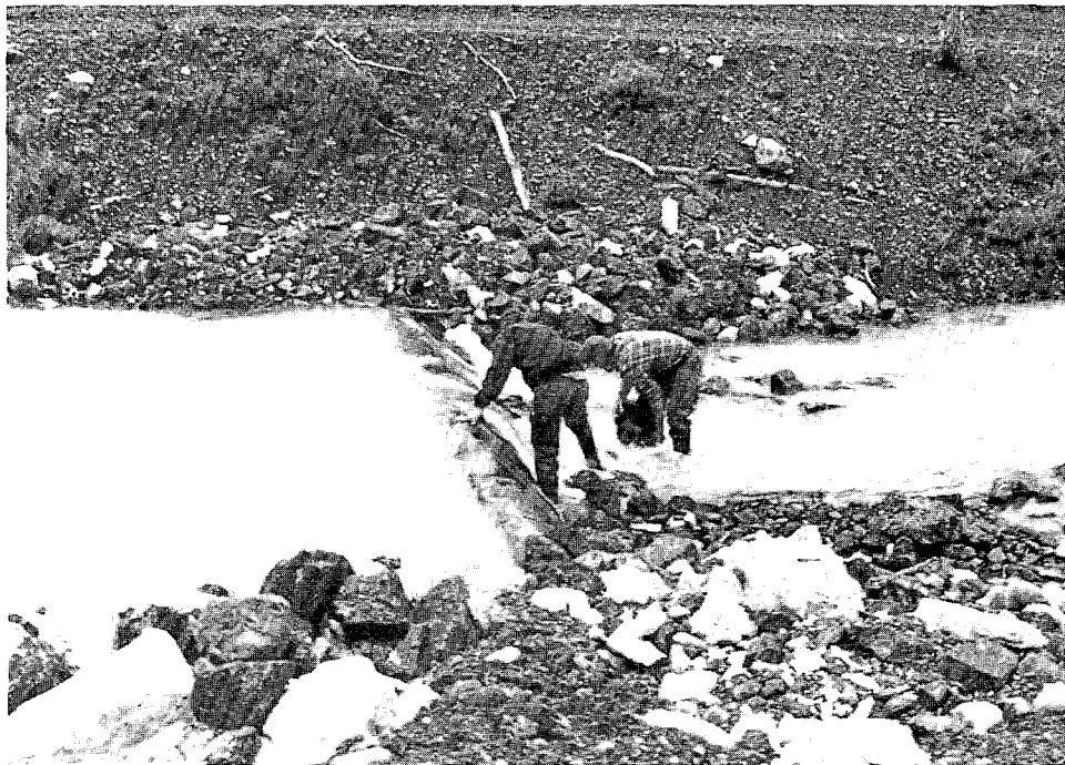
Plate 50. A notched log weir in the constructed spawning channel at the Martin River delta. When visited in 1993, several riprap rocks had washed below the notch, preventing fish from accessing the upper reaches of the spawning channel and other rearing areas. Regular inspection and maintenance is necessary for all instream structures.
