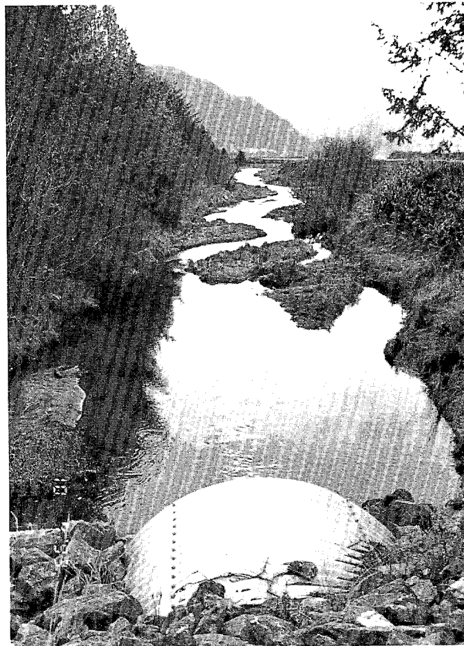
Plate 64. Besides correcting the perch, the arched culvert on Jordan Creek led to a more natural meandering channel downstream, by allowing the creek to cut its own path through the substrate (previously the channel was a straight run).
