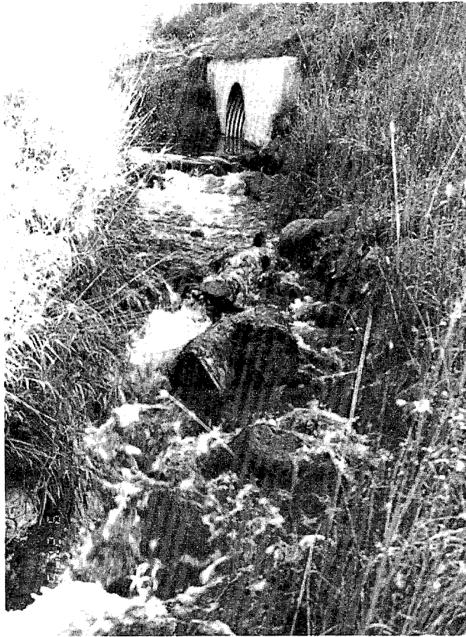
Plate 9. Rapids along the realigned loop section of Fire Creek as it exits the culvert north of the new highway interchange in North Eagle River (see Figure 5). The close succession of drop structures without resting space may be impeding fish passage through this section.
