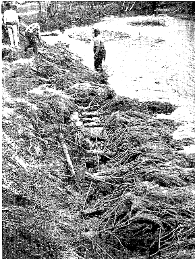
Plate 24. Volunteers installing a layer of donated Christmas trees on the eroding bank of Campbell Creek in 1992. Trees were anchored with a cable strung through the bases. Source: Fritz Kraus, ADF&G.
