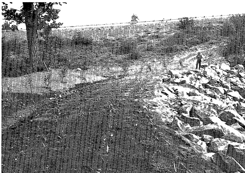
Plate 35. The west bank of Rabbit Creek just after replanting with riparian vegetation. Rooted willow cuttings are in the foreground; 4-6 ft. high transplanted willow trees in rear. 1988 ADF&G file photo.
