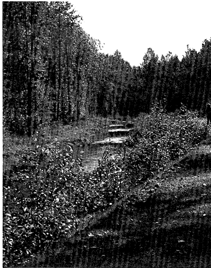
Plate 52. Box Canyon Creek rearing ponds near Seward, built as a series of small ponds separated by shallow riffle areas.
