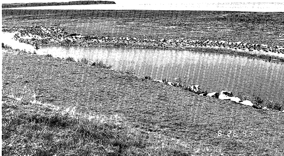
Plate 12. Coastal Trail mitigation project, consisting of an excavated pond and berm on the tidal mud flats in Anchorage. The brackish water pond receives stormwater runoff. Ducks primarily use the site as "loafing habitat," congregating on the bare berm.
