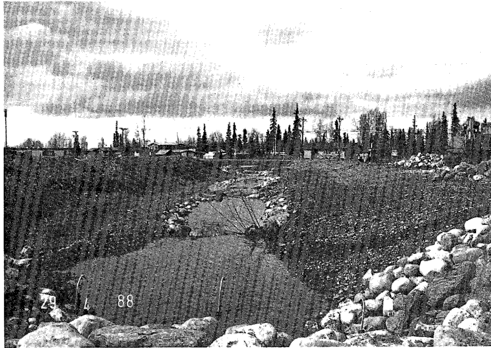
Plate 27. Realignment of Little Campbell Creek at Abbott Loop School. The new channel (700 feet long) included pool and riffle sequences to enhance fish habitat. 1988 ADF&G file photo.
