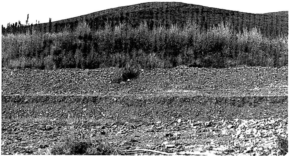
Plate 1. Independence Creek slope stabilization using dormant willows. Uppermost layer of overburden was planted four years earlier. Note high content of fine sediment in overburden stockpiles.
