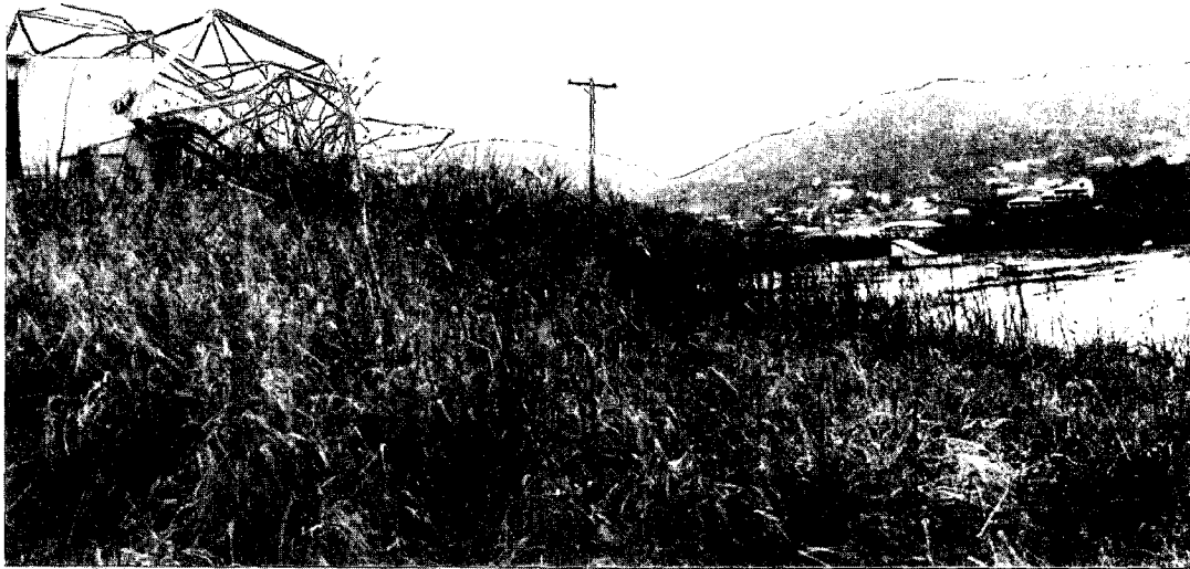
Figure 4-1. WSTX radio's tower collapsed during Marilyn. (Photo courtesy of Matt Stout)
