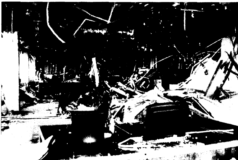
This photo depicts wind damage to the top floor of the Burger King World Headquarters building.
