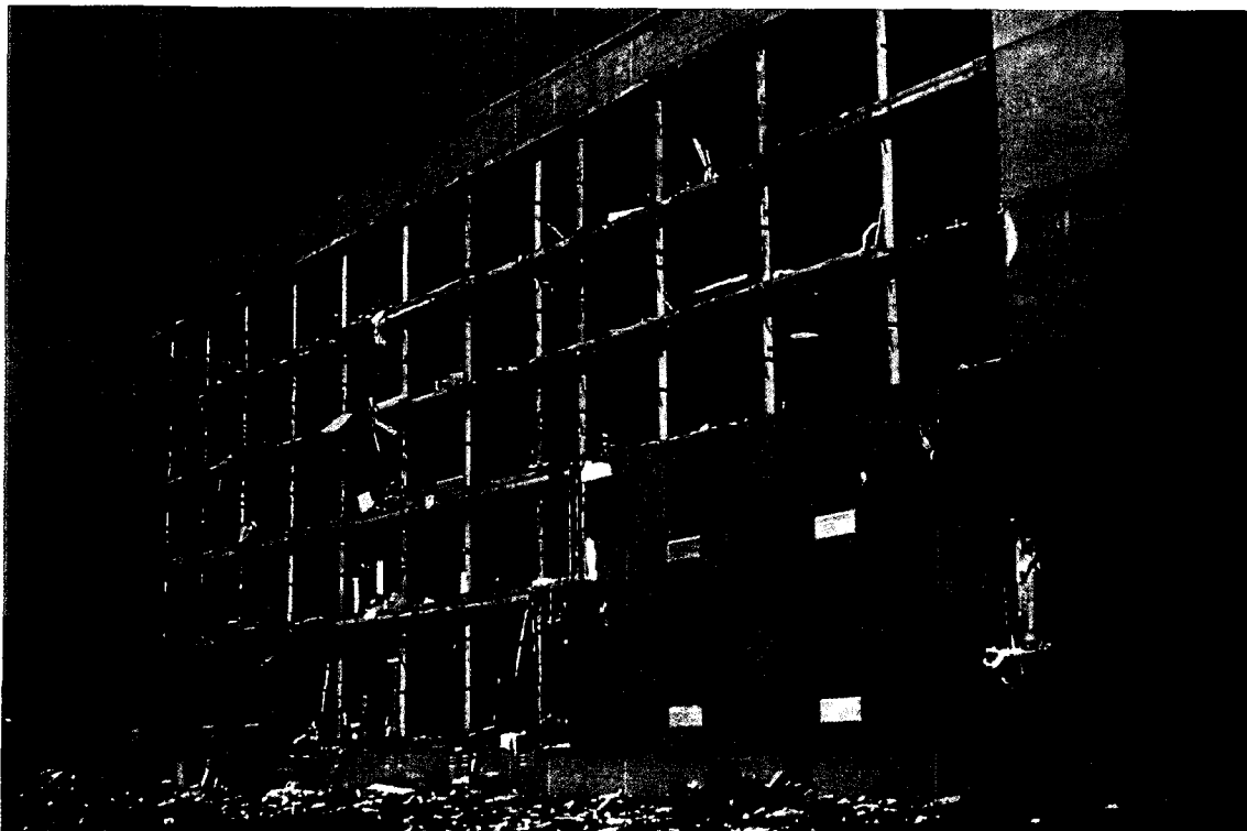
Intense winds associated with Andrew caused the shearwall to fail on the lee side of this multifamily structure.
