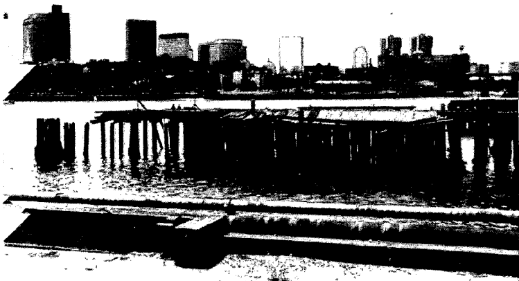
3-2 The deteriorated condition of bulkheads, piers, and pilings in many older cities is a major impediment to waterfront redevelopment.
