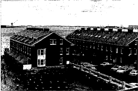
5-19 The new townhouses were constructed using flotation foundations and the units marketed as unfinished space.
