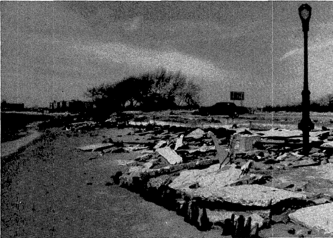
Coastal erosion at Plumb Beach, Brooklyn
