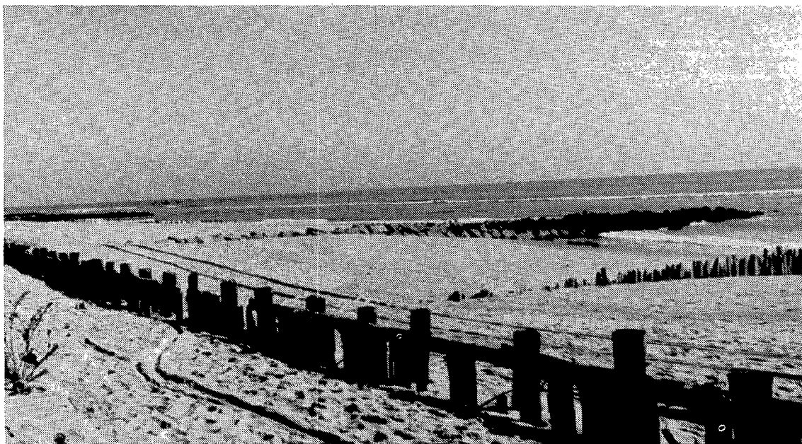
Shore protection jetties at Fort Tilden, Rockaway
