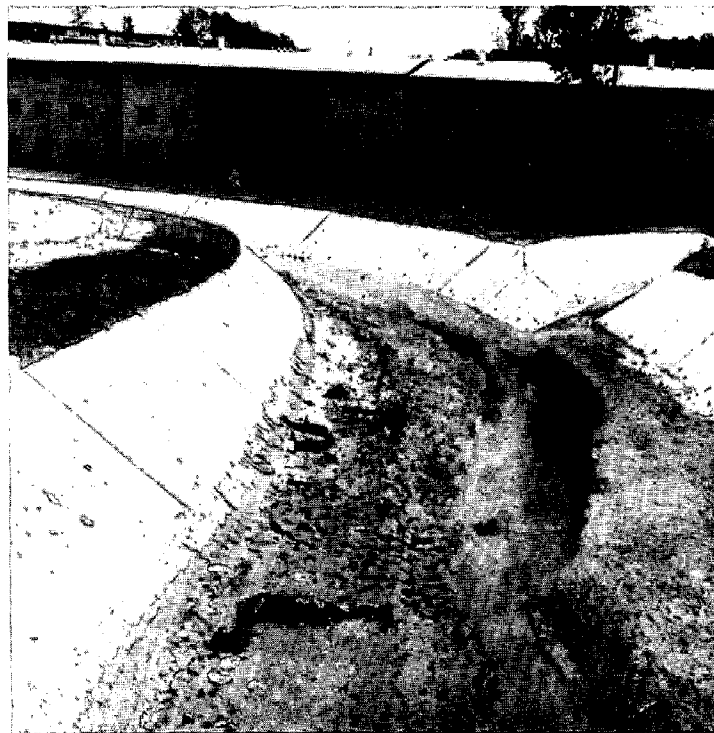
Poor planning and inadequate controls on urban fringe development can be costly to the community and to the natural environment. The photos show the effects of erosion, runoff, and sedimentation in Nebraska and Maryland.
