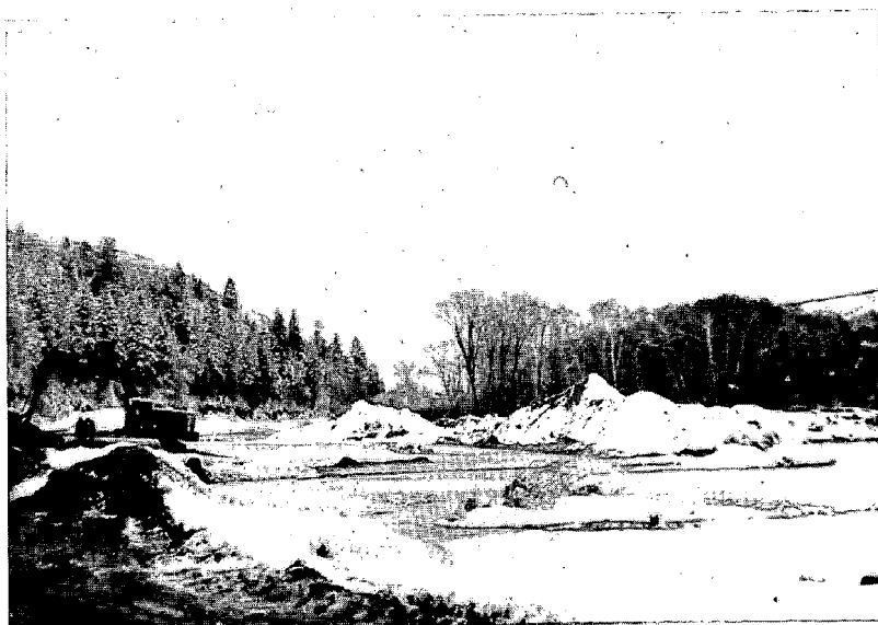
Piles of excavated material and other habitat disturbances resulting from access road construction below the Teton Dam site. Wildlife officials wanted the road located above the canyon rim to prevent covering the shoreline habitat, destroying fish spawning gravels, and causing downstream siltation in the river.
