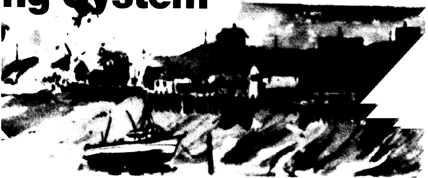
The 1946 tsunami roars into Hilo harbor . . .
