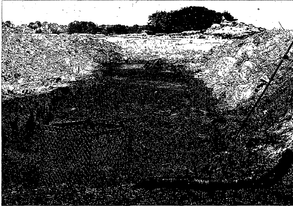
6-21. One of six ultimate disposal pits prepared in a clay area near the coastal town of Tregastel. Chemical stabilization has been considered for this material.
