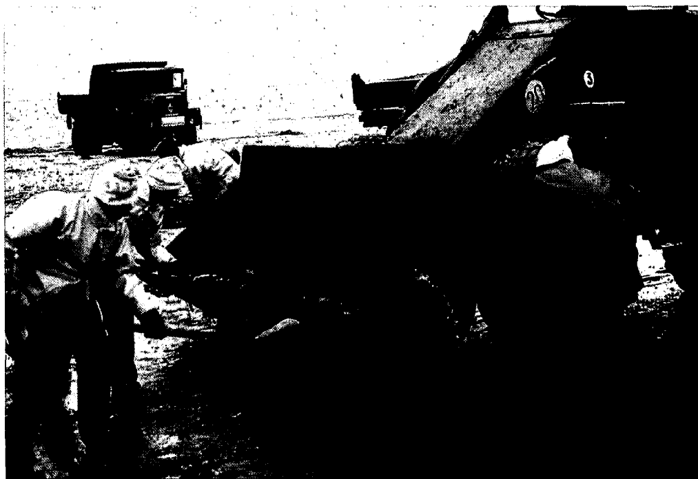
6-6. Workers scoop the oil into the loader bucket. The loader elevates it and dumps it into an Army dumptruck (shown in the background) for transport off the beach.
