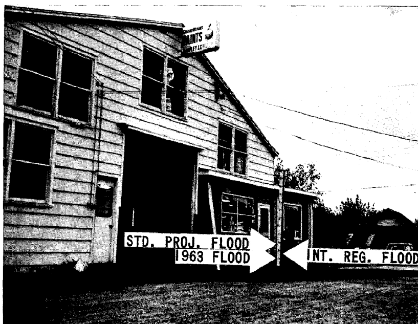
Figure 26. -- FLOOD HEIGHTS AT HAWLEY LUMBER YARD
