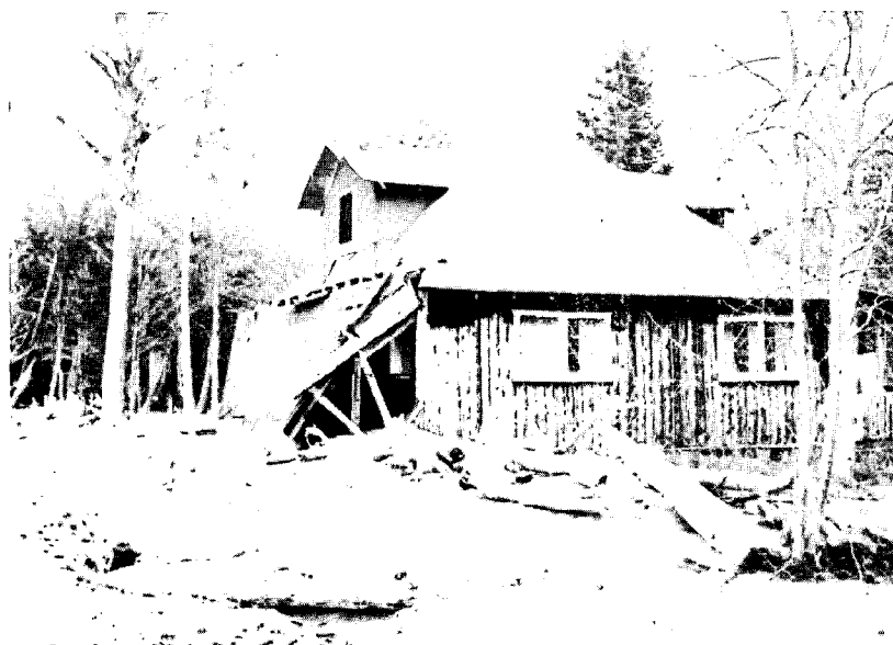
Figure 31. -- PROPERTY DAMAGE - REACH NO. 4
