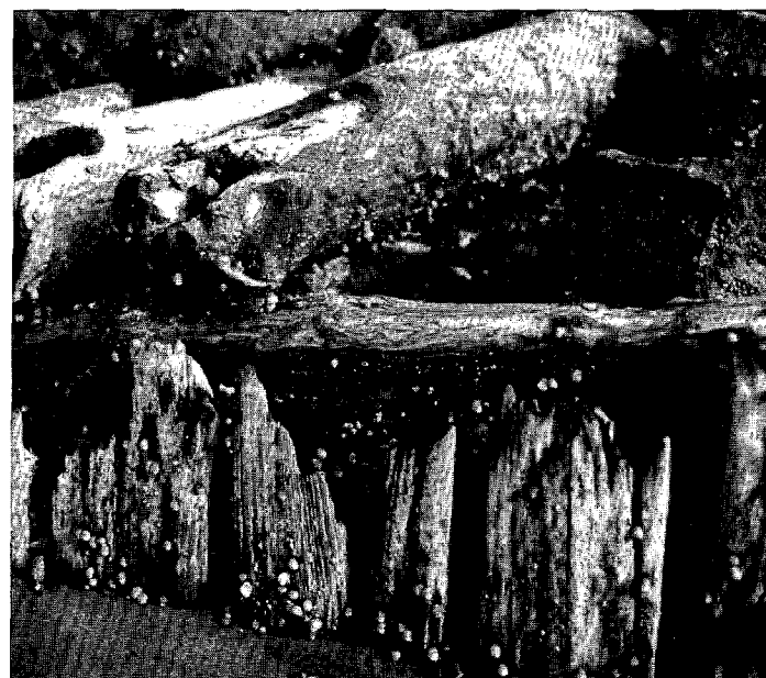
Fig. 3.8. Early 19th century wharf and jetty details. A , Cribwork of Gunnison's Wharf; B and C , Plum Island breakwater, built in 1831. Note trunnel construction.
