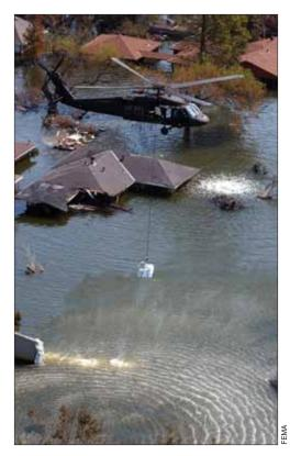
surrounding neighborhoods.<sup>99</sup> When Hurricane Katrina led to the breaches in the levees, the lack of access roads atop the levees resulted in very significant increases in time and cost to repair the damaged areas.
