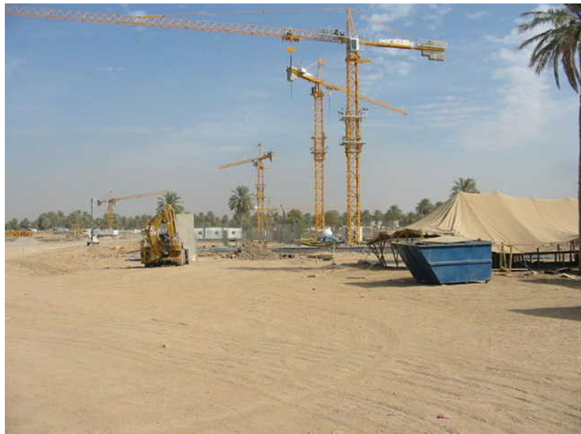
Four Tower Cranes
