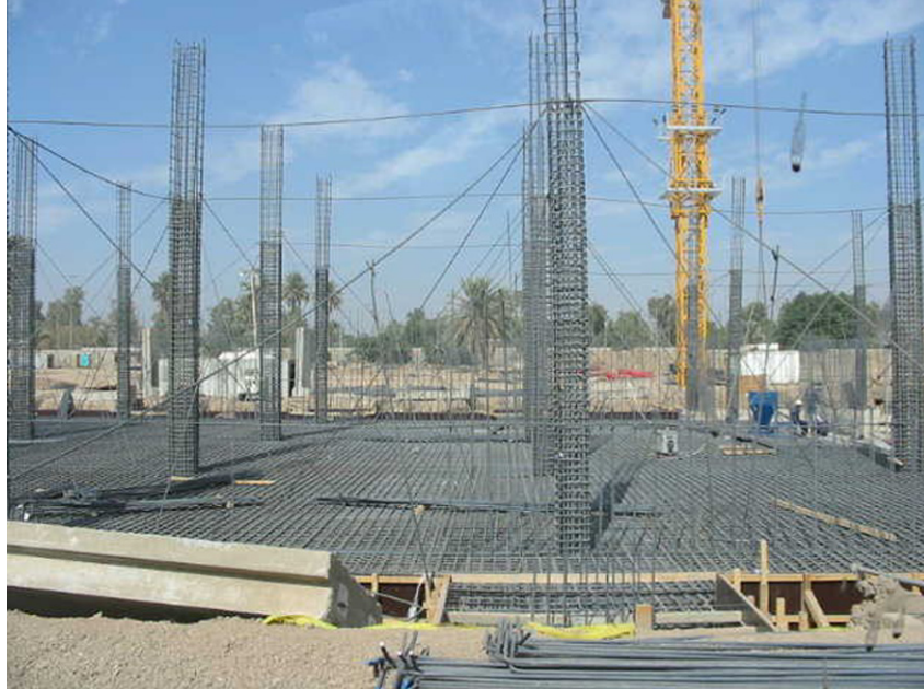
Embassy Baghdad Construction 11/06/2005
