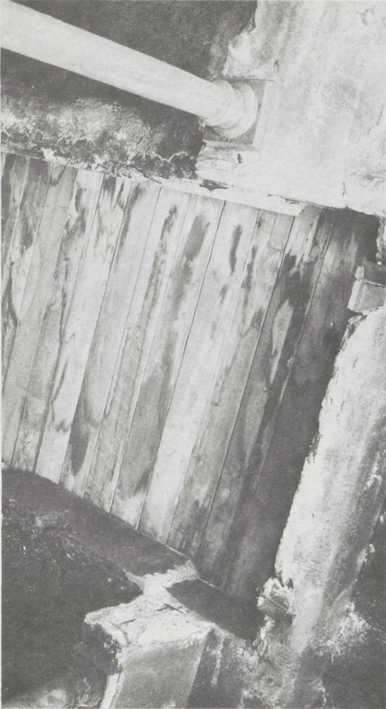
Decay of existing wood decking over old elevator shafts.
