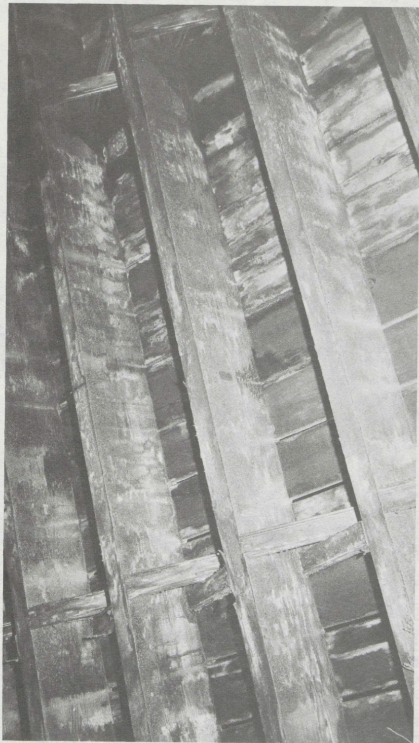
Decay of existing wood decking over old elevator shafts and support wood deck for ticketing office.
