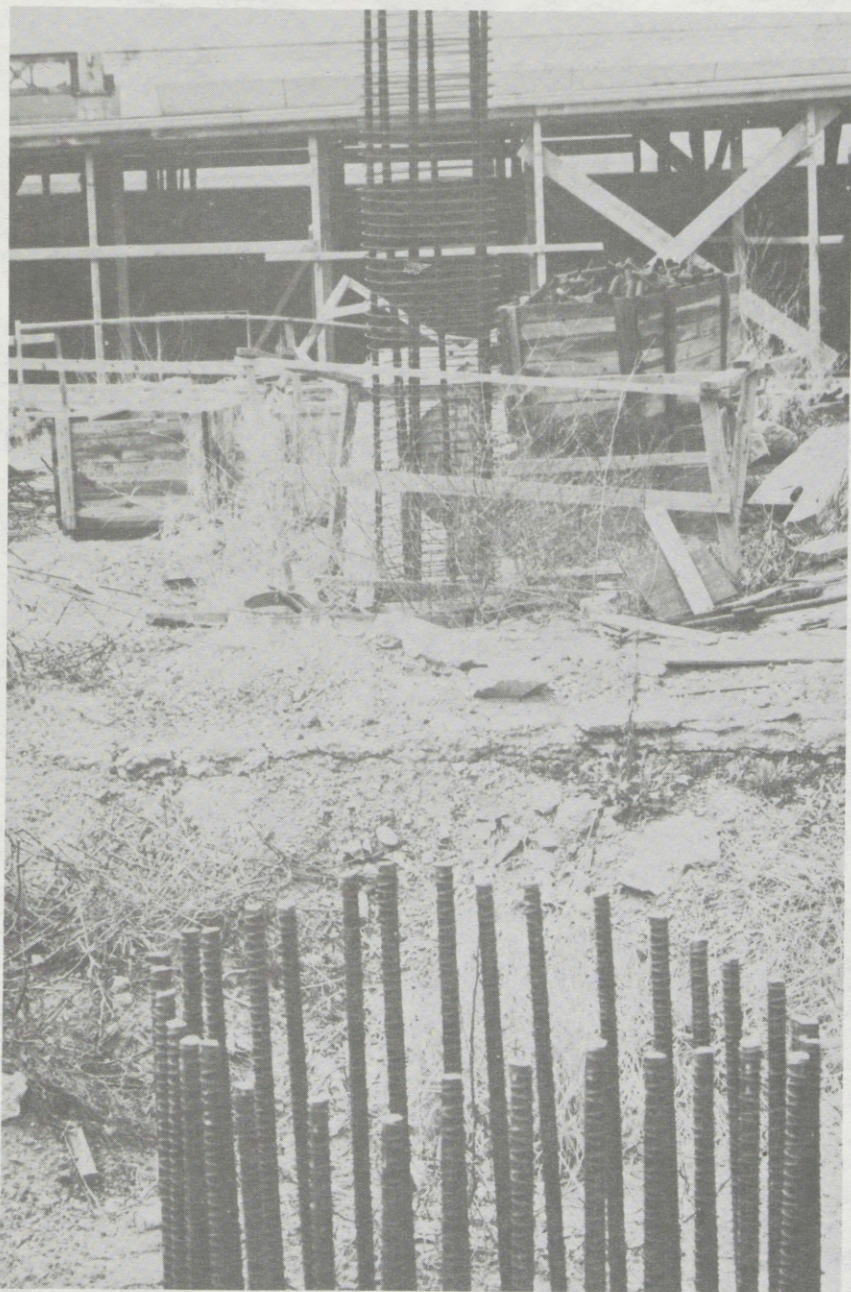
Exposed reinforcing of uncompleted parking garage. Reinforcing has begun to corrode, rust and deteriorate in some areas, due to exposure to the elements.
