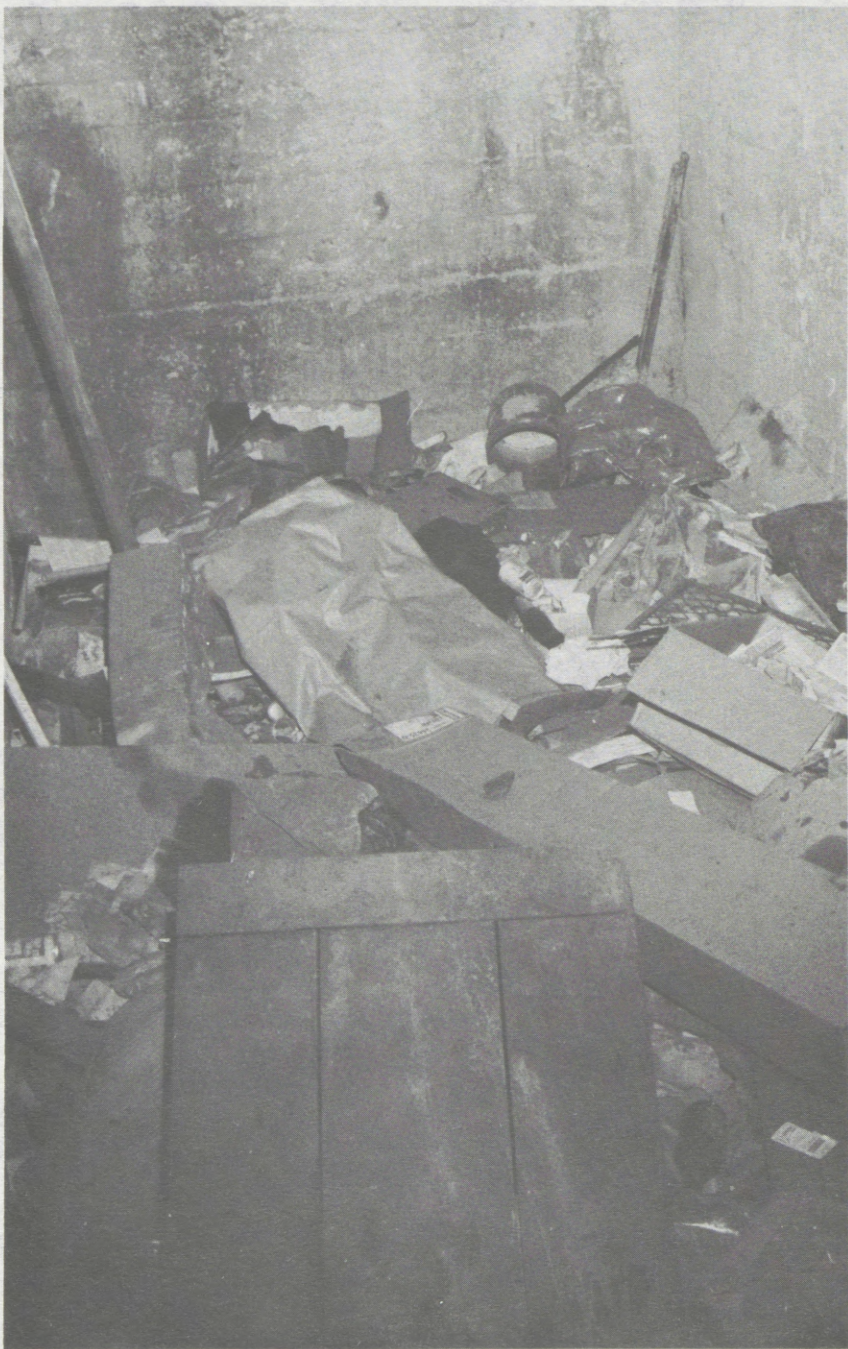
Debris in abandoned elevator shaft (several shafts are in similar condition). These shafts are covered by wooden platforms—fire hazards as they are located above temporary wood walkways to train platforms.
