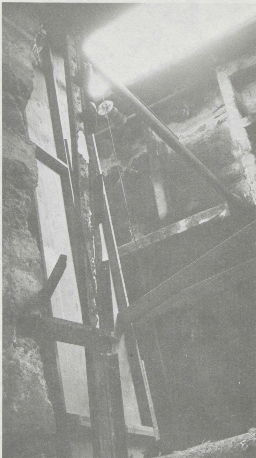
Decayed wooden platform—termite ridden and rotted—supported by temporary 8" x 4".
