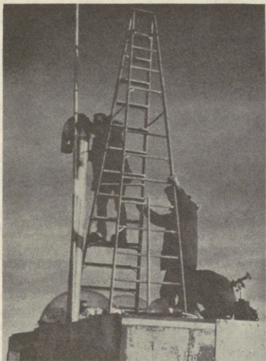
Construction in progress at the NOAA Global Monitoring for Climatic Change Station at the South Pole is shown. (Department of Commerce photo.)
