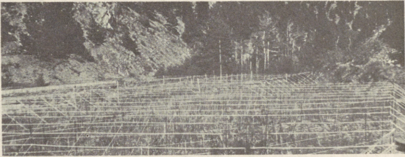
The new incoherent scatter radar antenna installed by the NOAA Aeronomy Laboratory at Sunset, Colorado. (Department of Commerce photo.)
