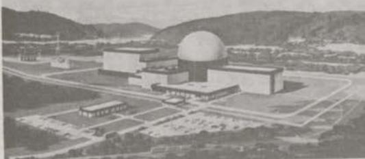
*Construction progress on the Fast Flux Test Facility (FFTF) near Richland, Washington. The 400 megawatt thermal reactor is a liquid sodium-cooled, fast flux reactor designed specifically for irradiation testing of fuels and components for the liquid metal fast breeder reactors. Bechtel Power Corporation is architect-engineer; Advanced Reactors Division of Westinghouse Electric is lead reactor designer.*
