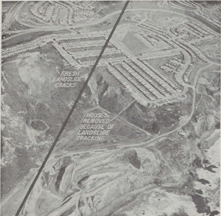
FIGURE 4.—Land-use planning. Houses should not have been built astride the 1906 break of the San Andreas fault or on potential landslide developing in crushed rock along the fault zone. Photograph along San Andreas fault, Daly City, Calif. Heavy line is position of 1906 fault break; dotted line is approximate boundary of fault zone.
