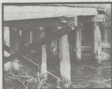
Deteriorating bridge pilings on Ottertail River Bridge. Bridge provides access for visitors using the refuge for recreational purposes.
