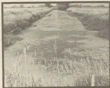
Silt filled ditch affecting water management program on refuge.
