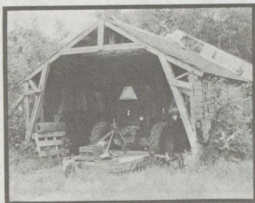
Storage shed for heavy equipment. Reconverted building originally designed for another purpose.
