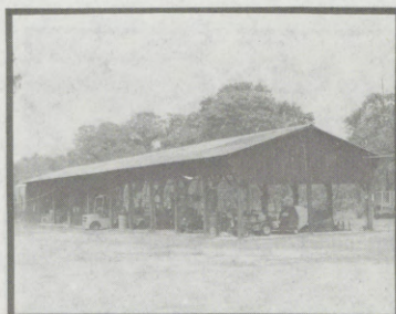
Deteriorating equipment shed.
