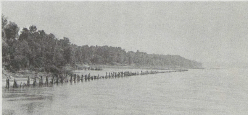
A wandering Missouri River has been made narrower and swifter with the use of wooden pile dikes. The dikes tend to deflect river current toward the center of the channel; silt accumulates behind the dikes, creating new land and a narrowed river.
